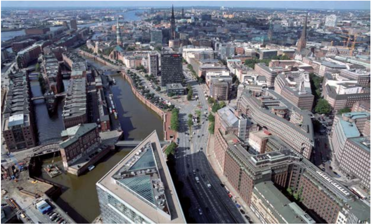
Aerial view of Speicherstadt (left) and the Kontorhaus district (right)
