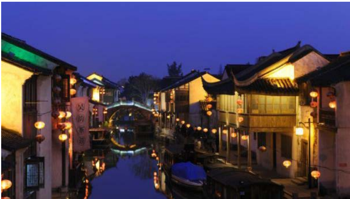
Shantang canal conservation zone
