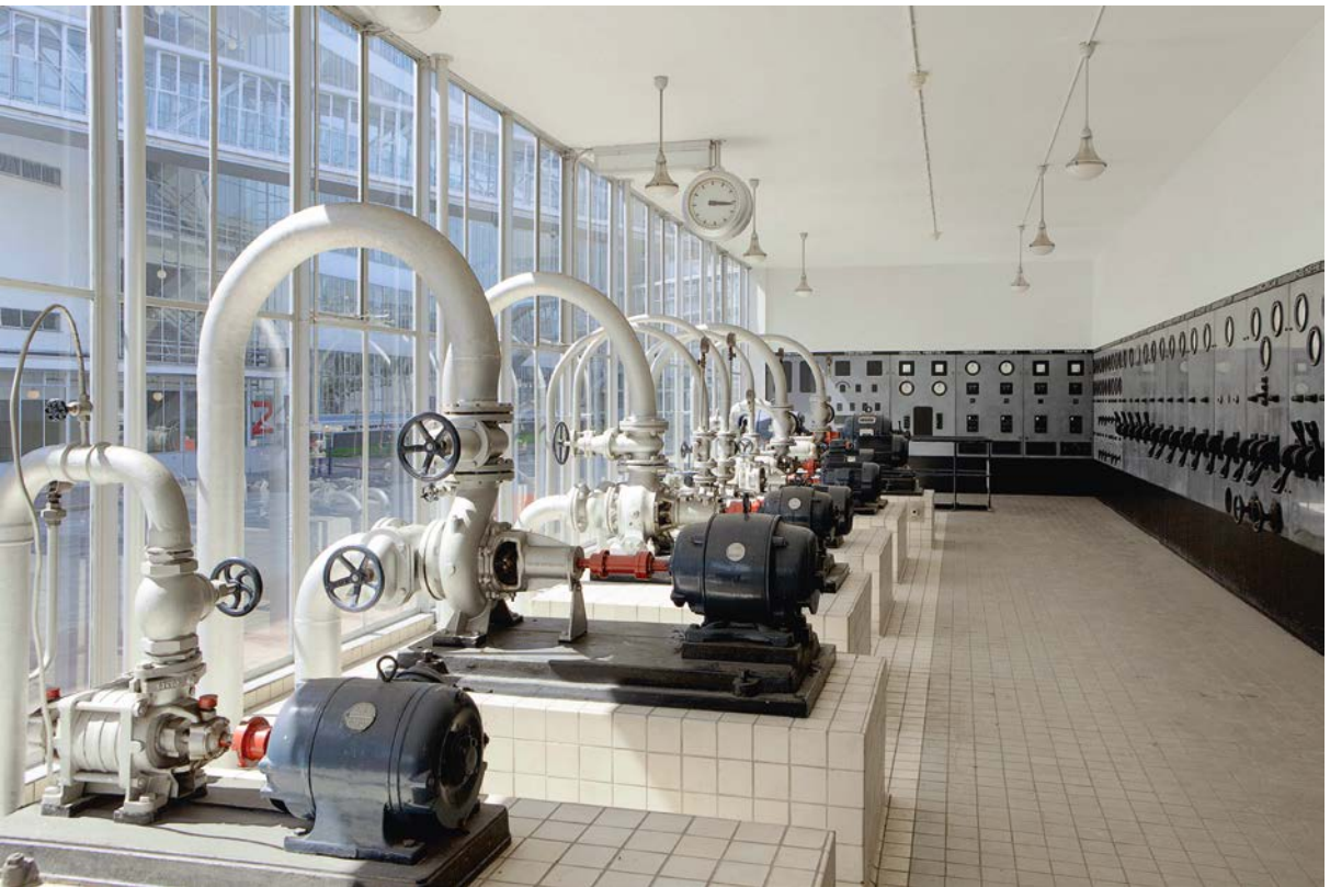
The boiler house
