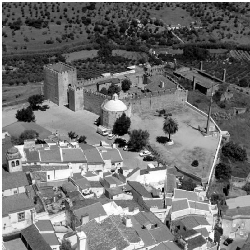
The Castle of Elvas – aerial view
