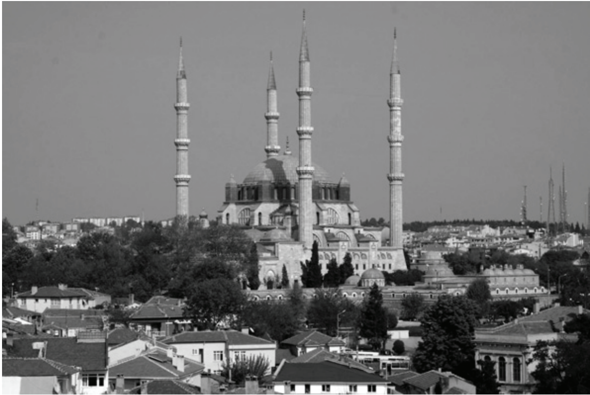
General view of the nominated property
