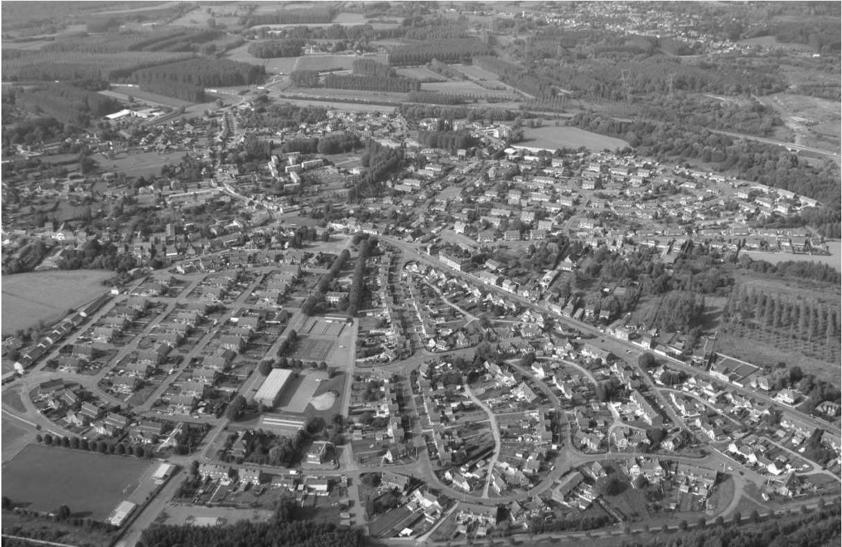
Aniche mining company - Worker estates of Sainte-Marie, Lemay and Pecquencourt
