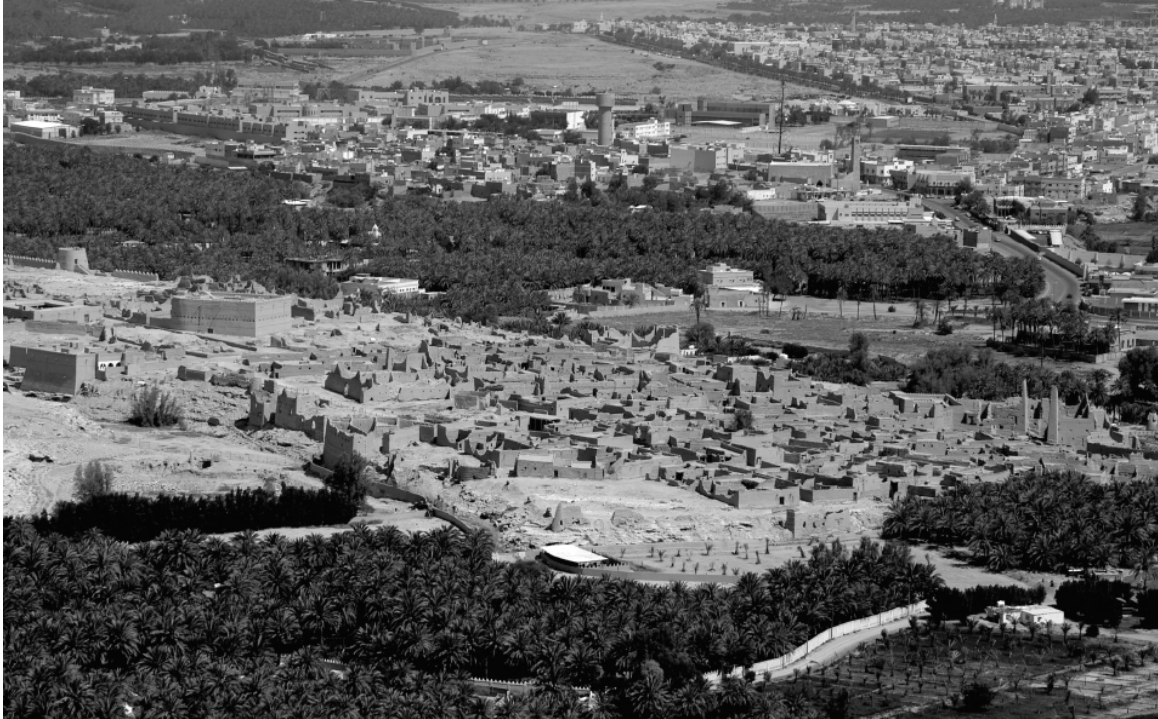
General view of the nominated property
