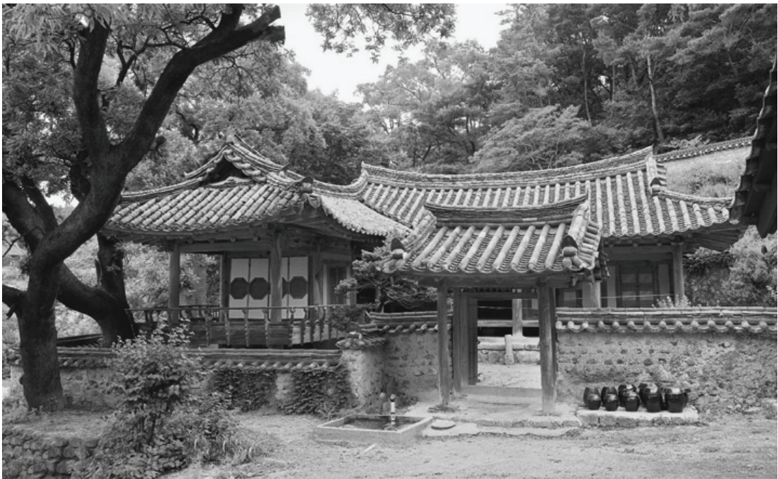
Yangdong Village, Simsujeong Pavilion
