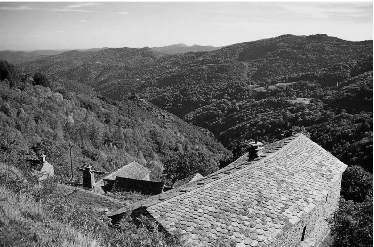
Roof in shell-shaped slates
