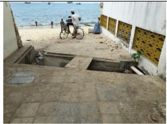
The beach access from the narrow walkway has missing paving
