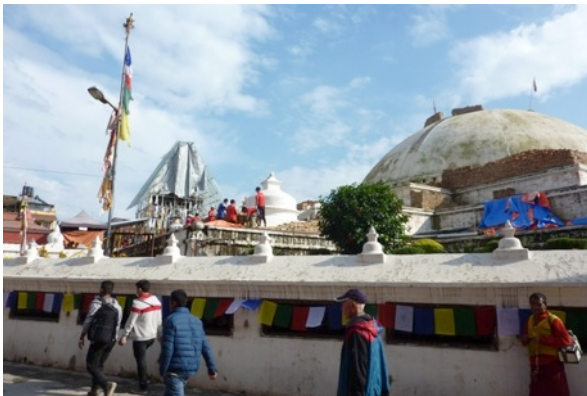
The top portion of the Bauddanath stupa was damaged and has since been dismantled for repair.
