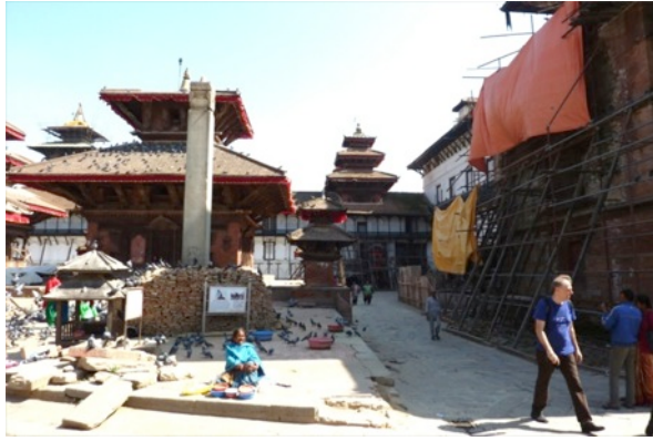
Temporary propping in place to support damaged structures (Degu Telegu on right)
