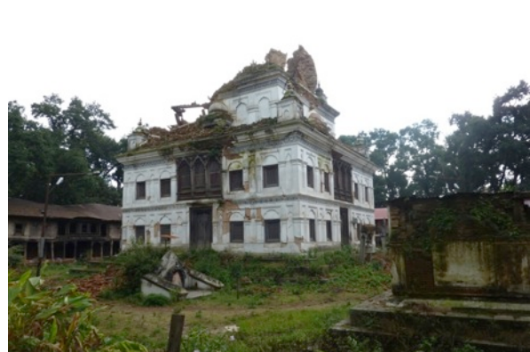
Collapse of dome to Vishwarupa temple on top of hill
