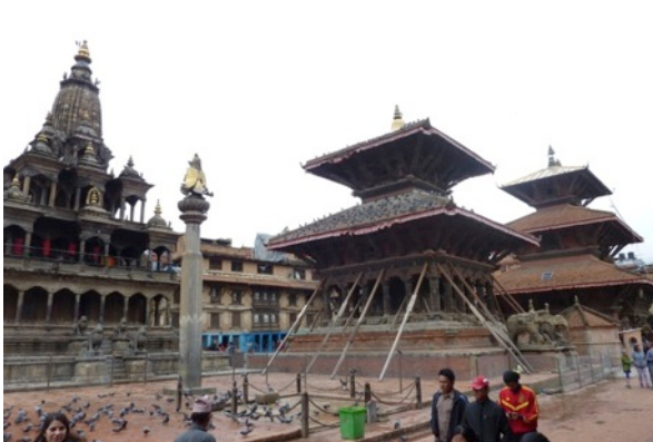
Propping of temple in Patan Durbar Square. Most temples in the square survived.
