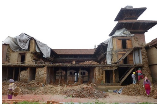
Rear wing of museum damaged and in process of being demolished.
