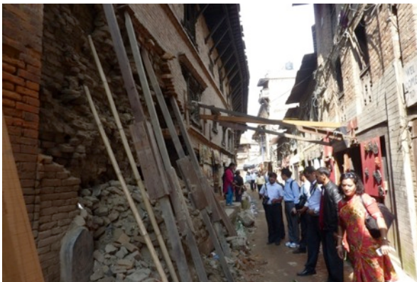
Damage to wall around Peacock window
