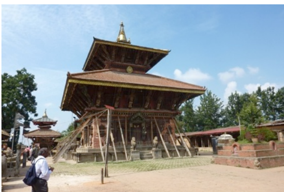
Changu Narayan temple is propped. Corner brickwork has already been relayed. Laxmi Narayan Temple destroyed (left of main temple)
