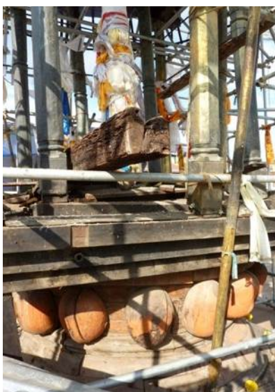
The timber crown and canopy elements are to be repaired and re-erected on top of the stupa
