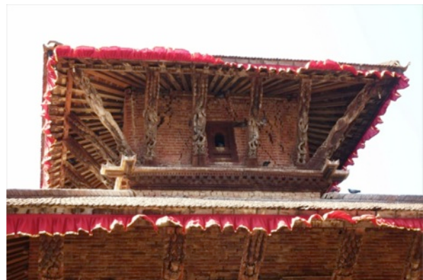
Loose bricks in upper tier of temple provide a hazard to visitors
