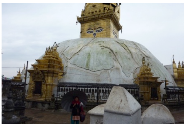
Cracks in dome of Swayambhu stupa were sealed to protect the stupa during the monsoon rains. They are to be repaired during the dry season.
