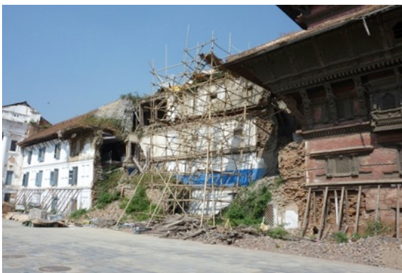
Serious damage to and partial collapse of nineteenth century portions of palace (facing Nautale Durbar)
