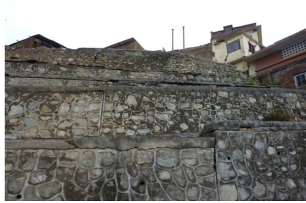
Sattals collapsed around the edges of the hilltop. There is some evidence of movement in the retaining walls constructed to stabilise the hillside.
