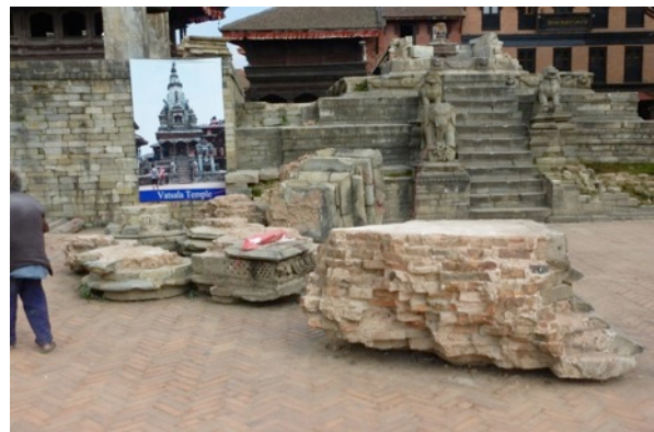
Batsala temple, which had been repaired using cement, collapsed.
