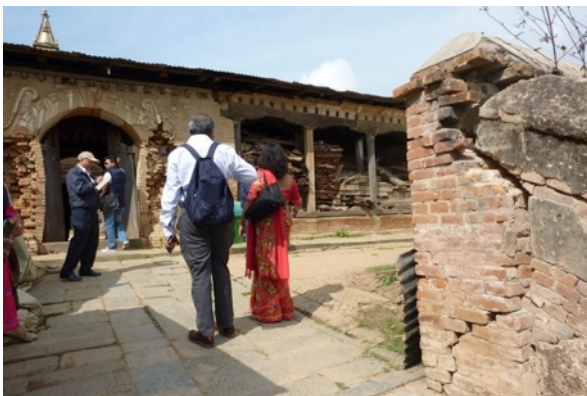
Stairs and entrance gate to temple complex damaged. Upper floors of the sattals were severely damaged and were subsequently demolished. Materials are stored on site
