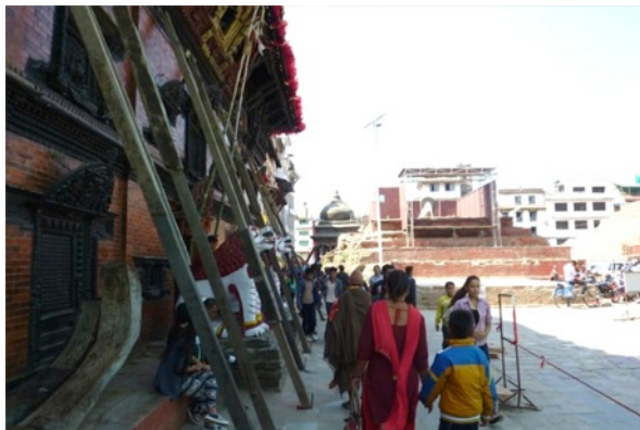
Temporary propping of Kumari Ghar (left) and protective hording around surviving lingum on tiered base of destroyed temple enables daily rituals to continue.
