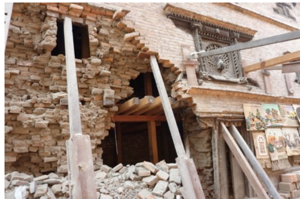
Damage to wall around Peacock window
