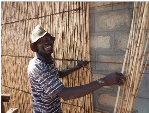
The new perimeter wall and the current installation of reeds to hide the cement blocks
