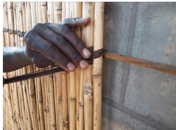
The new perimeter wall and the current installation of reeds to hide the cement blocks
