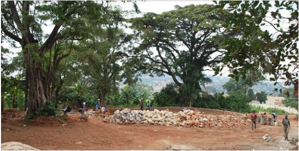
Slab under construction to exhibit the burnt steel
