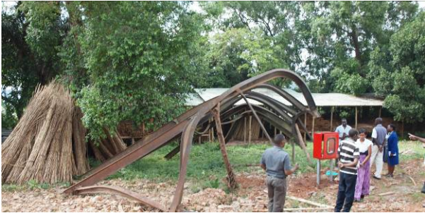
Remains of the previous roof structure
