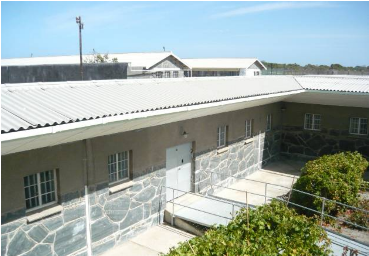
Main building of maximum security prison
