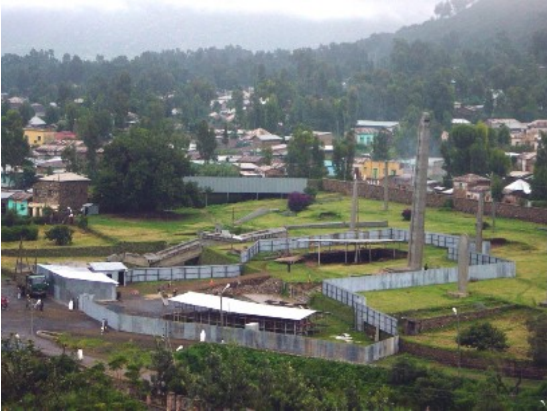
Aksum Construction site: general view
