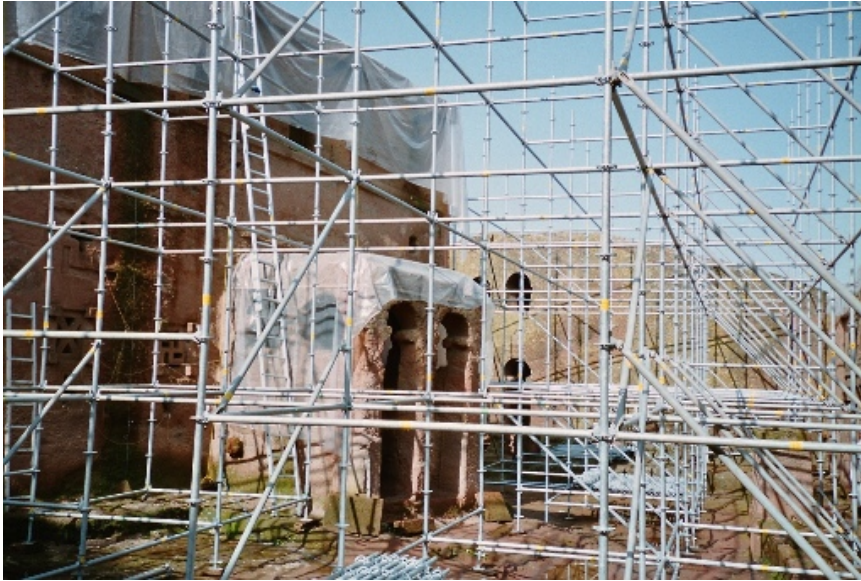
View of the Scaffoldings at Biet Mariam
