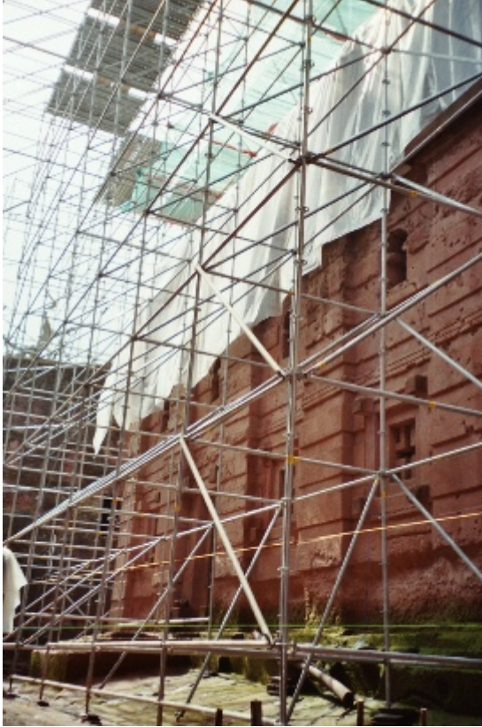
View of the scaffoldings at Biet Amanuel
