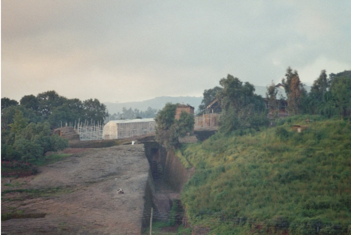
View of the shelters construction work site showing Biet Mariam
