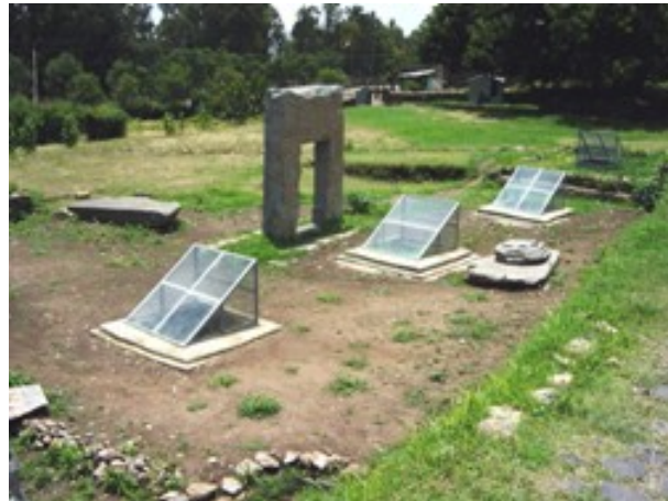
Ventilation/protection elements for the underground galleries (World Bank Project)
