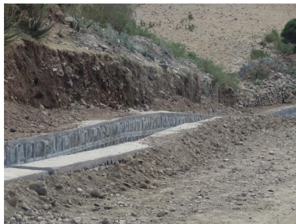
Figure 17. Close-up photograph of the new storm water gutter on the road to the Tombs of Kaleb and Grebe Meskel. (Author)
