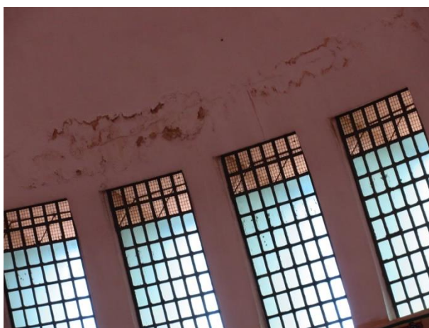
Figure 24. Water damage to the inside of the main dome of the Church of St Mary of Zion (Author)
