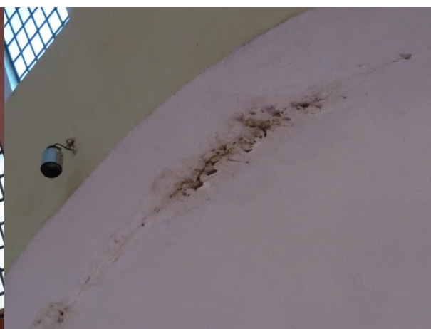
Figure 25. Water damage to the inside of one of the vaulted apses of the Church of St Mary of Zion (Author)
