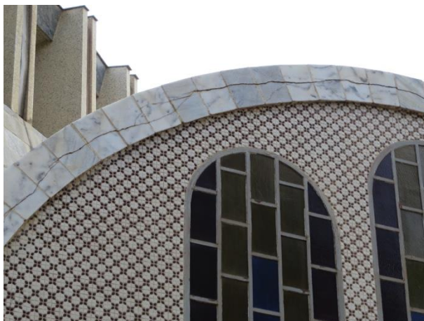
Figure 22. Cracks along the circumferences of the vaulted apses of the 1957 Church of St Mary of Zion. (Author)
