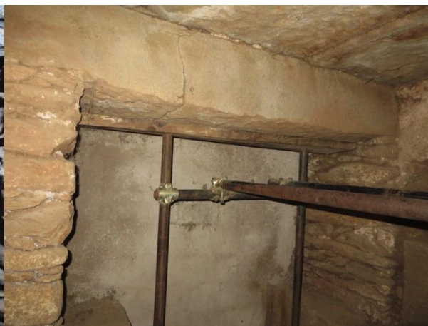
Figure 7. Temporary scaffolding supporting the historically cracked lintels in the Mausoleum. (Author)
