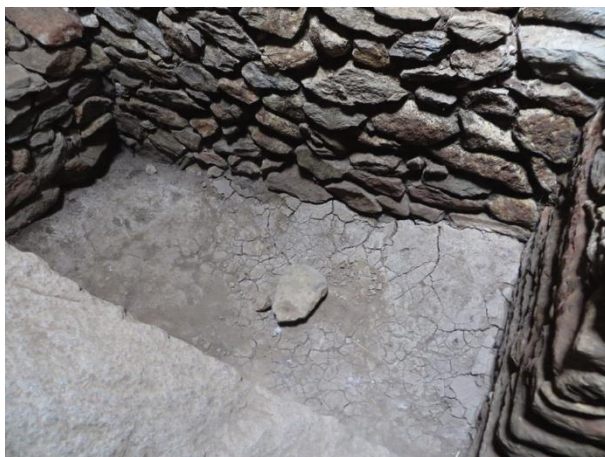
Figure 6. Evidence of rainwater ingress in the end chamber of the Mausoleum. (Author)
