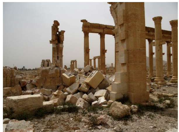
Most of the collapsed stones of the Triumph Arch still on site
