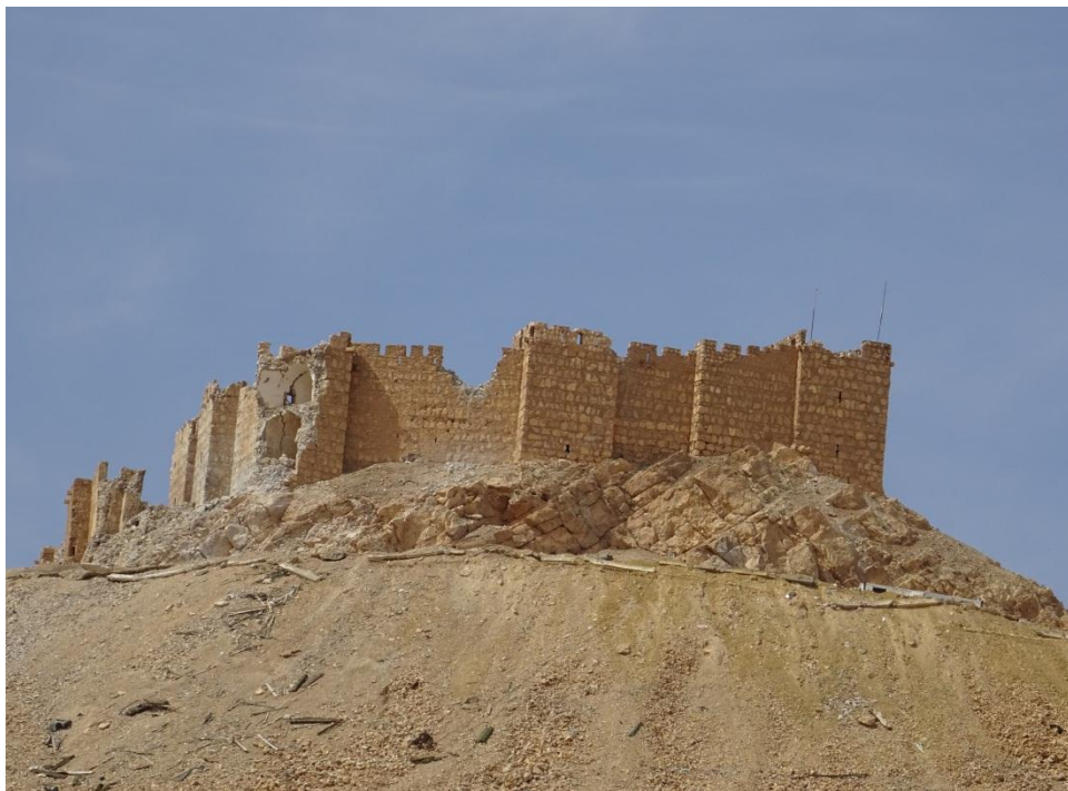
Close footage showing the top of the walls partially collapsed in several locations of Castle of Fakhral-Din al-Ma'ani
