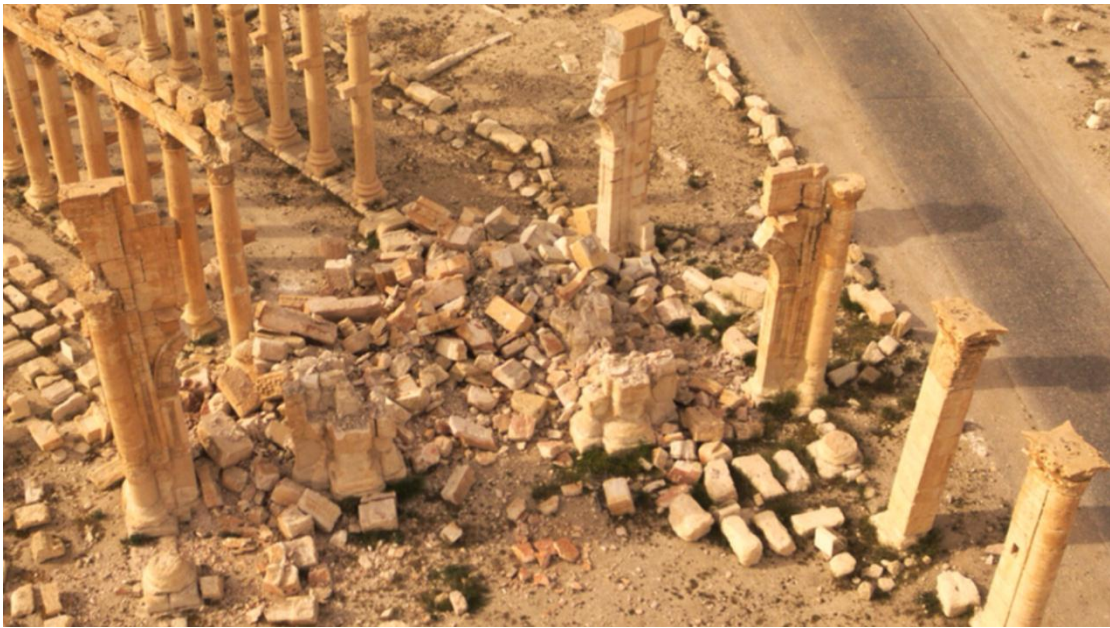
Aerial Footage showing the damage of the Triumph Arch
