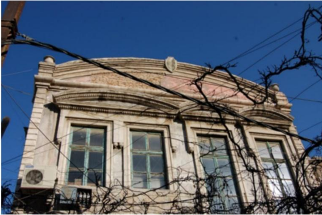
The North Facade before damage
