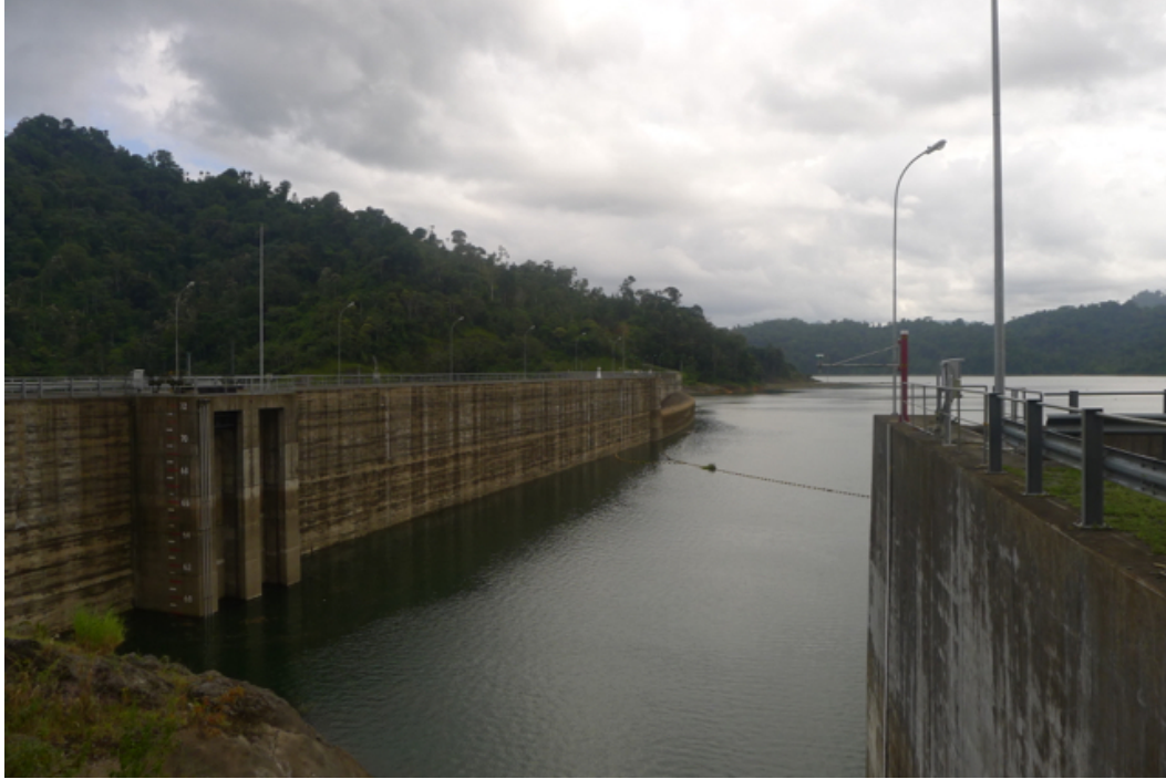
CHAN 75 dam and part of reservoir. 14 January(© Robert Hofstede).
