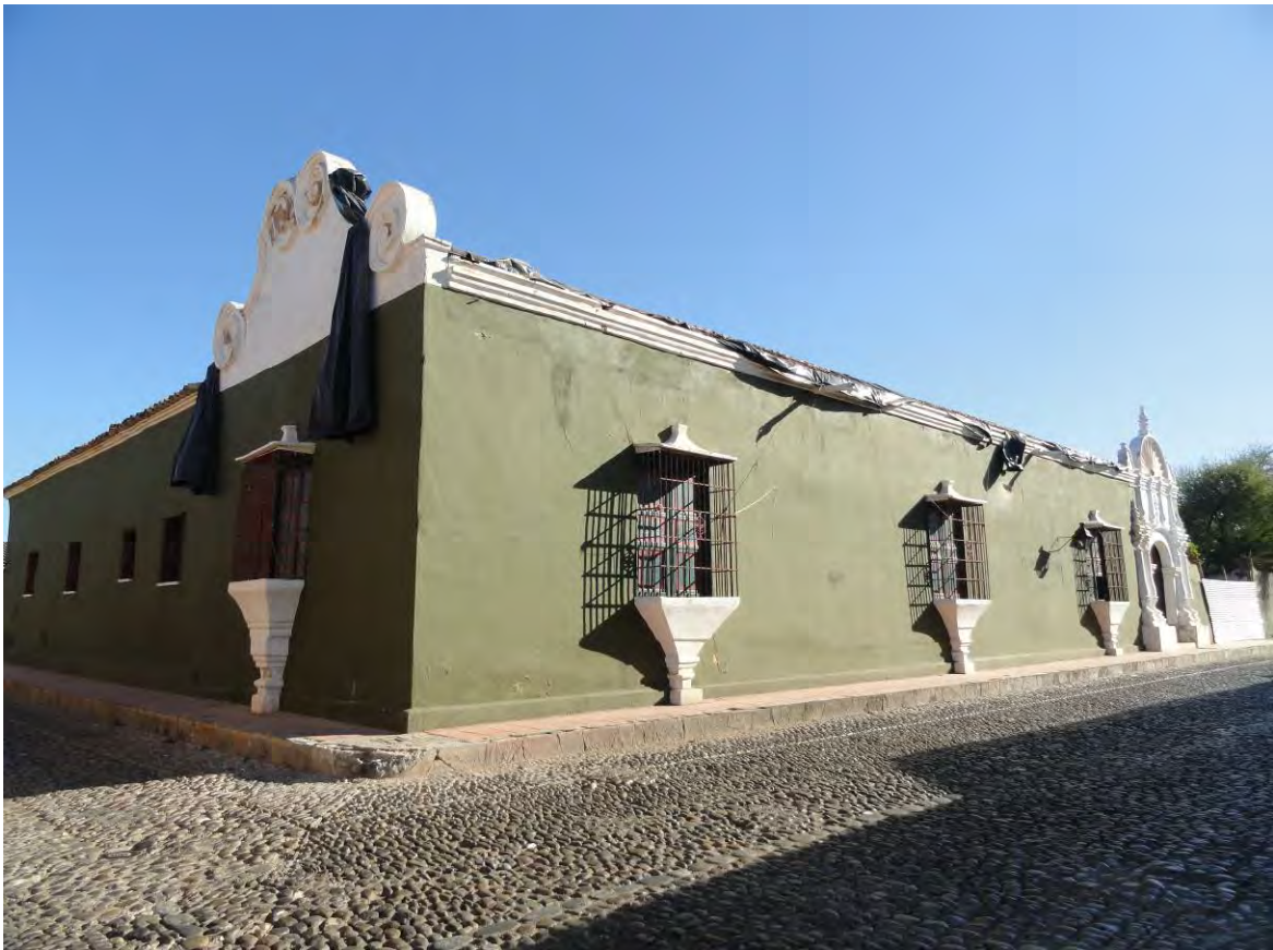
Photograph 07. The same House in 2011 with temporary plastic roof covers
