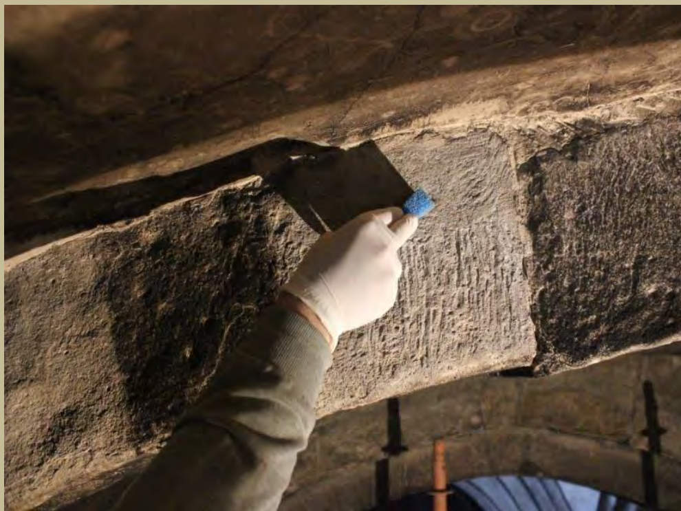
Photo: The process of cleaning of stone surface with sponge
