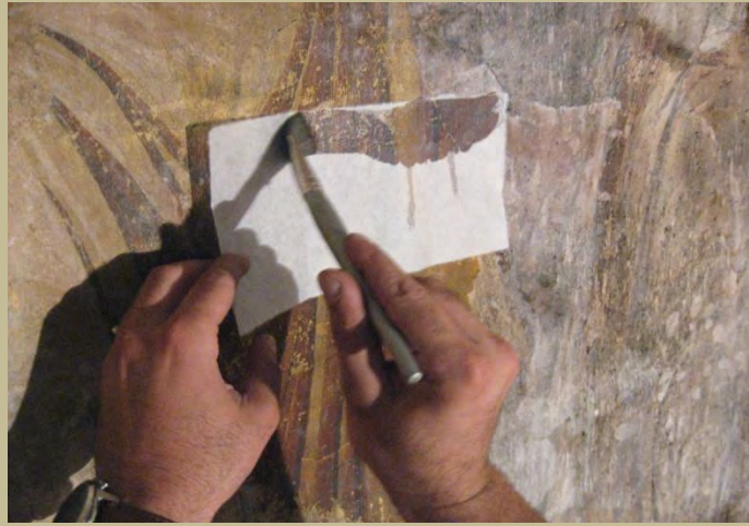
Photo: The process of strengthening of color layer
