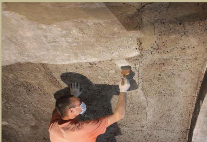
Photo: the process of cleaning of stone surface
