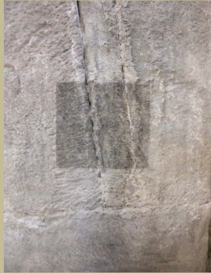
Photo: The process of cleaning of stone surface in the sanctuary
