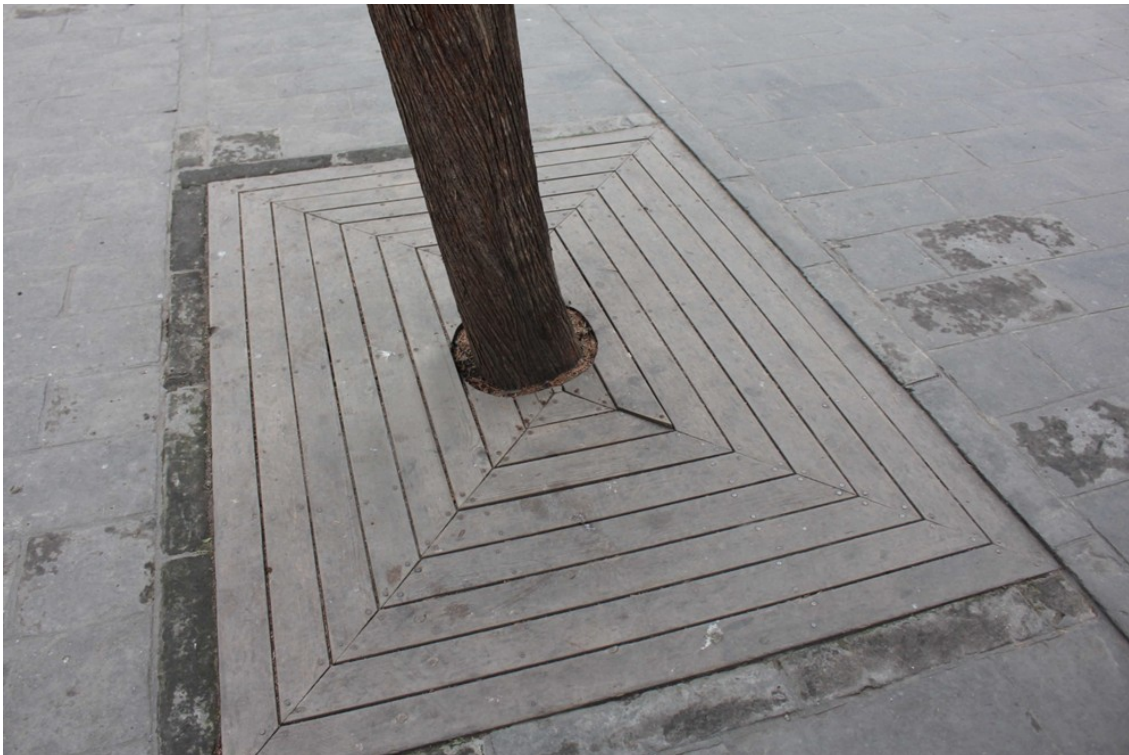
Wooden tree guard, allows adequate soft area around the tree
