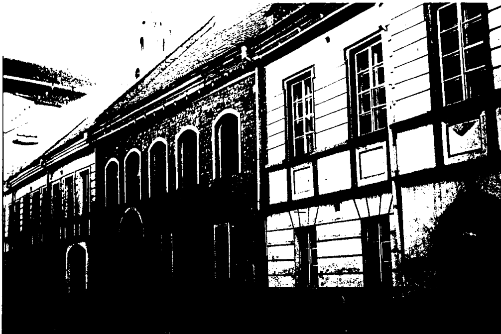
fig. 5. The houses in Pilies Street 13 and 11. Of the three Neoclassical facades, the one in the center was restored to its Gothic looks. The dark bricks are original, the light ones modern.
