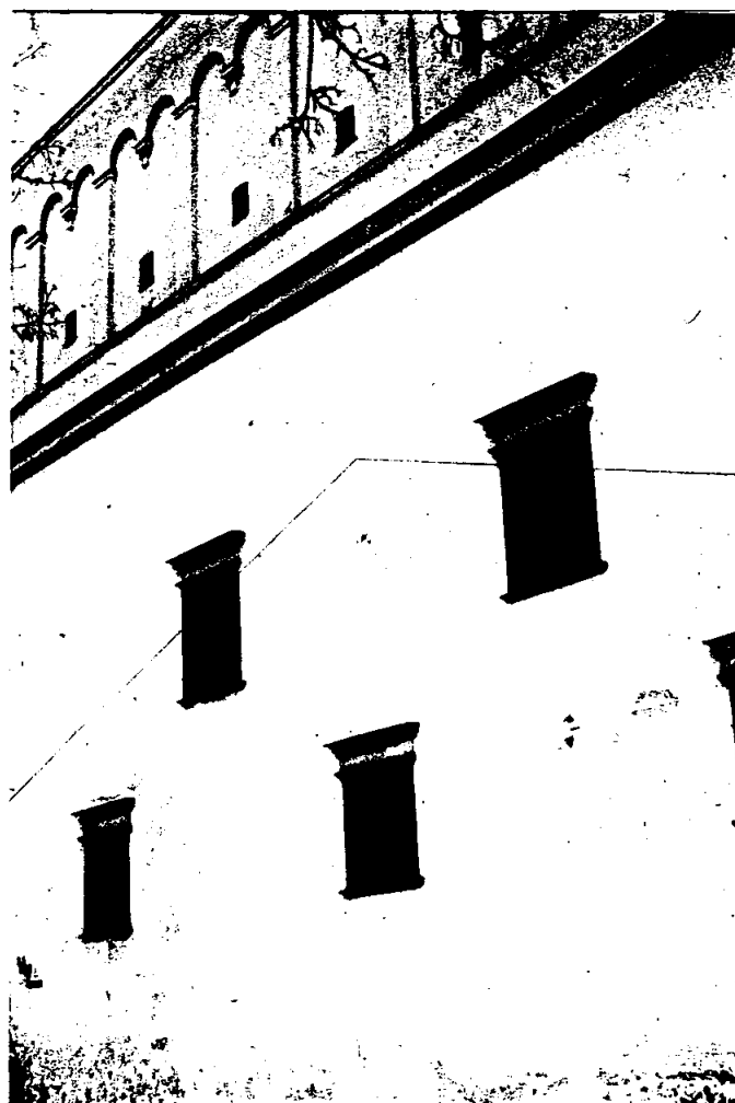
fig. 4. The restored gable of the Arsenal. The line in the facade indicates the preserved part of the wall. The window frames are of concrete, with small fragments of original sandstone.
