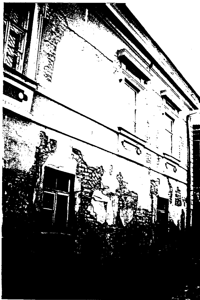
fig. 6. Building archaeological research openings on the facade of the house in Bernardinu 6. The decision of the restoration is not made yet.
