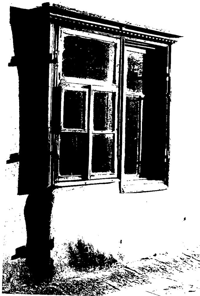
fig. 10. A beautiful but neglected wooden window in Bernardinu 10. Some of the windows of this house have already been changed into new ones of inferior quality, possibly because oil paint and putty for restoration are not available.
