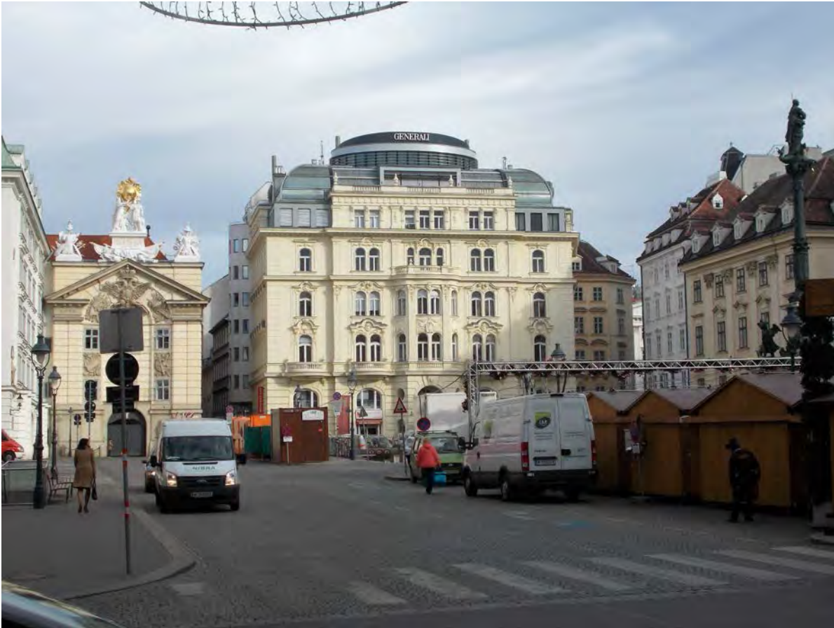
10 - Modification of the roof of the historic building adjacent to the Bürgerliches Zughaus, Platz am Hof
