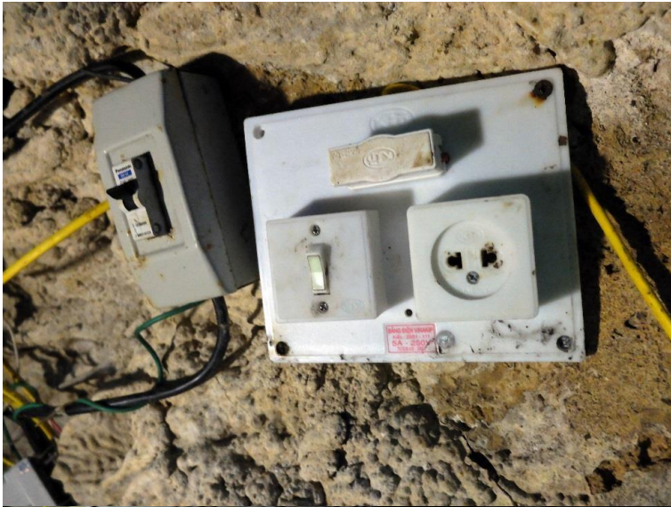
9. Power switches in cave located above the level reached by flood water in wet season
