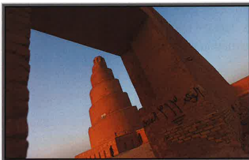
Fig,3 Painting Great Mosque walls
