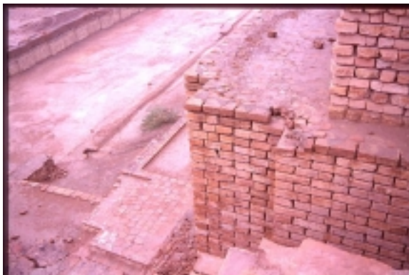
Figure 11 Detail of lower walls of the ziggurat, showing areas that need constant maintenance and repair, particularly after heavy rains.
