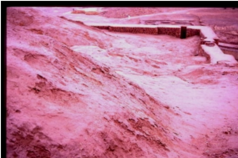
Figure 7 The corner of the mud brick mount, showing outlets for drainage.
