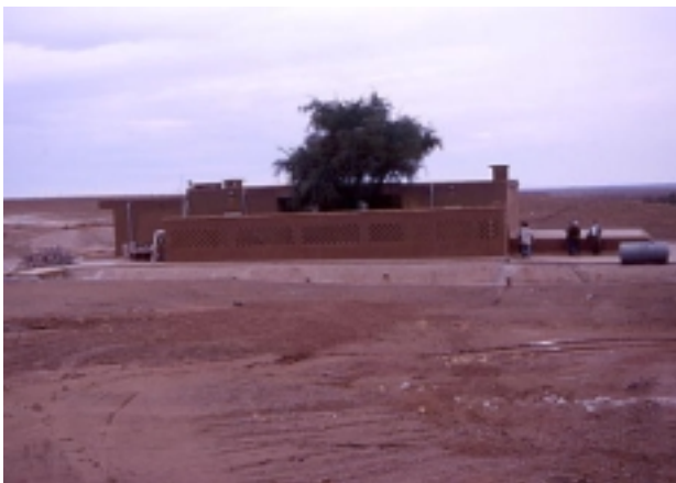
Figure 17 A small modern construction that has been repaired and partly rebuilt as a service centre for site work. It includes, e.g., studio facilities, a meeting room and storage.
