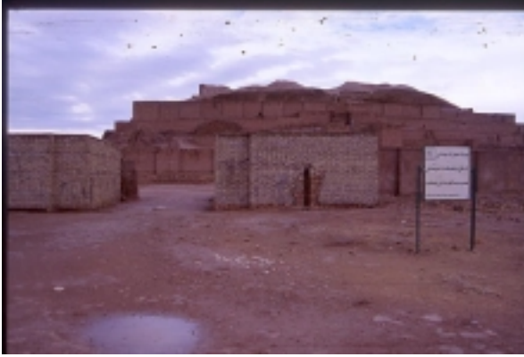
Figure 12 Entrance in the inner wall, showing the cement brick walls rebuilt some three years ago to contain the original mud brick structures.
