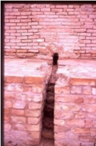
Figure 10 Detail of drainage outlet
