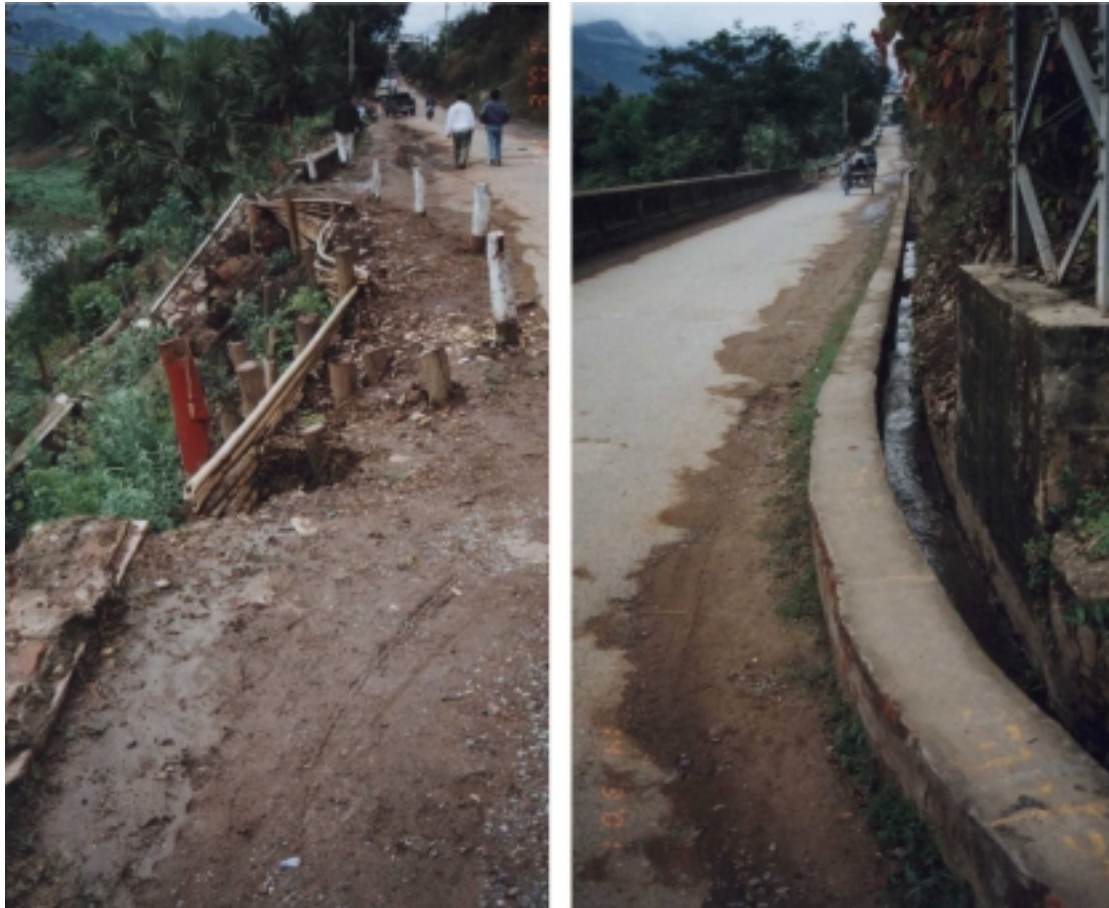
Figure 4 (left) shows the site of the main failure, and how it affects the road. Figure 5 (right) shows the drainage ditch adjacent to the rock face (also shown in Figure 1). The wet area along the verge of the road shows where rainwater has lain, unable to escape via the ditch.
