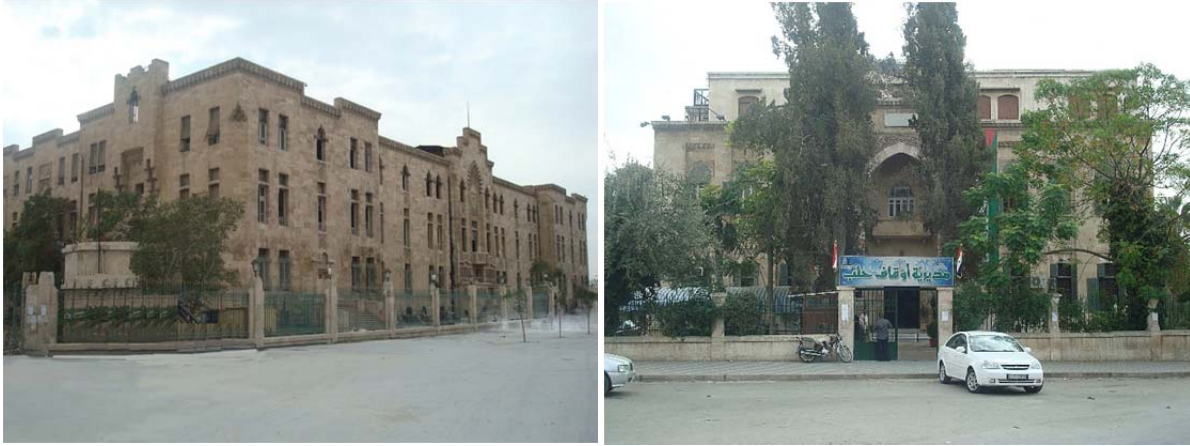
Aleppo, Architecture of Modernity buildings, Colonial and Post-colonial period, (© A. Soufan, 2010)
