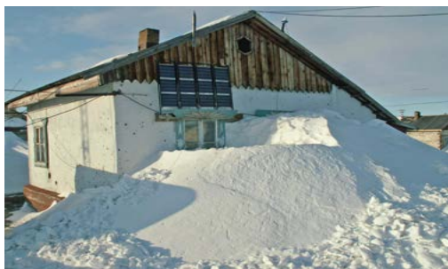
Fig. 9. Solar panel is used on the base Ushakovskoe in the spring and autumn. Using of wind turbines may be the most effective way to generate electricity during the polar night.
