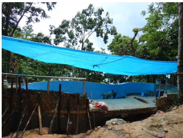
Construction of Infinity pool at Sitio Panaguman
