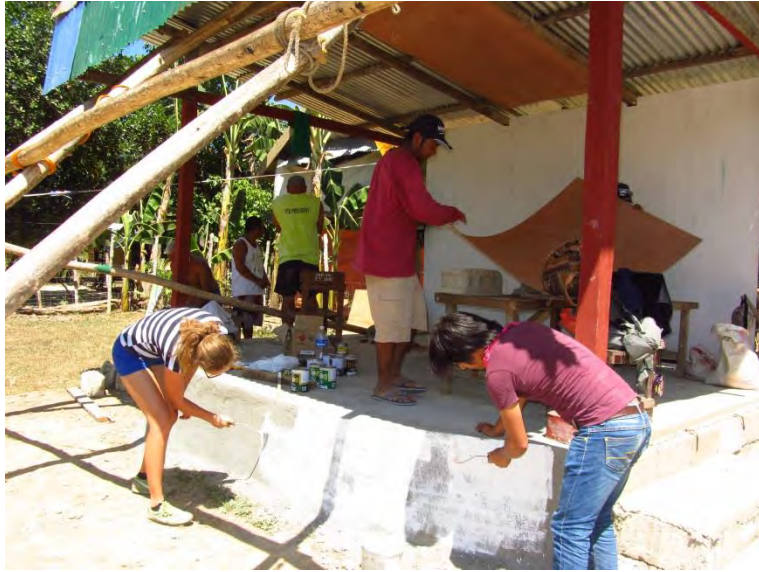
Sitio Bayatao School Stage construction
