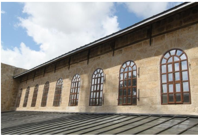
Figure 12: View of the completed windows
