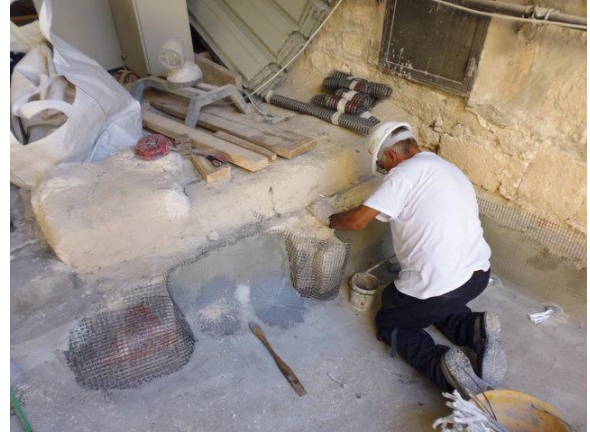
Figure 22: net of glass fibers immersed in a cement matrix
