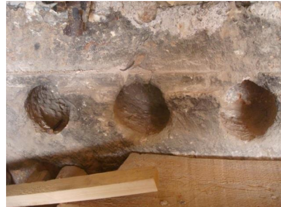
Figure 2: holes excavated in the walls during Justinian's time
