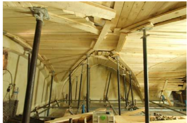
Figure 20: Lateral propping
