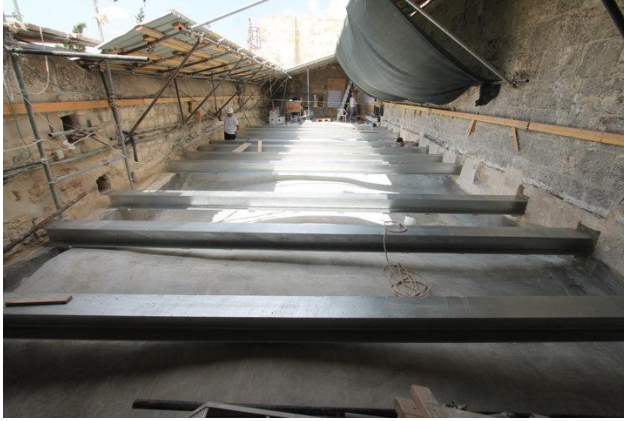
Figure 24: Beams connecting both façades
