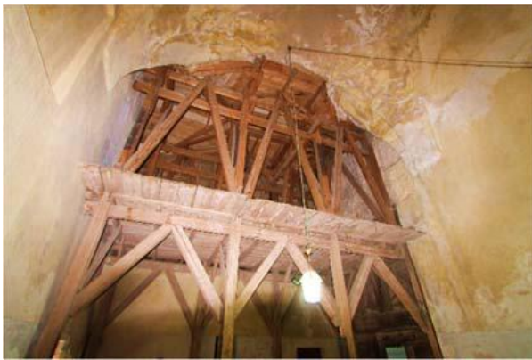
Figure 19: Central propping
