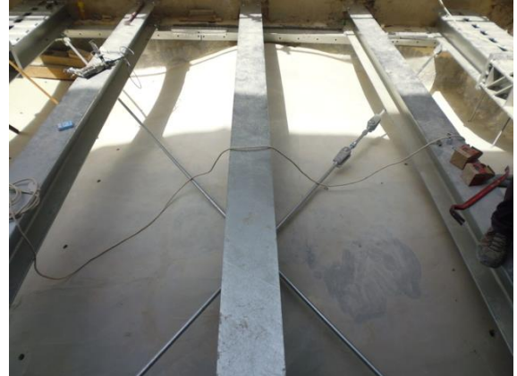
Figure 25: Bracing system
