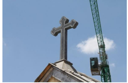
Figure 11: New crosses installation
