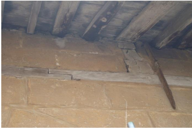
Figure 1: stones above the present wooden sleepers at the higher level
