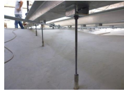
Figure 29 Hanging rods
