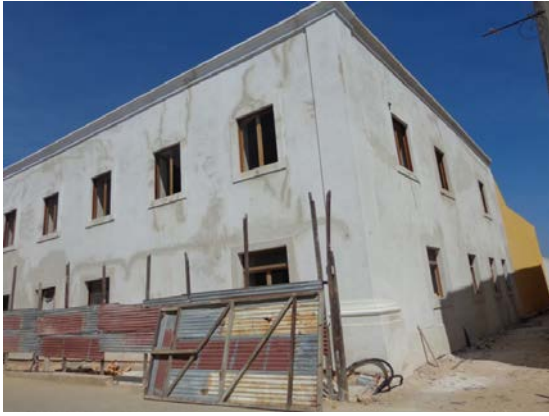
Fig. 3 Trading Depot Hotel, in the final stage of restoration
