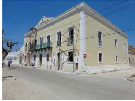
Fig. 4 Restoration of the Municipality building, in progress
