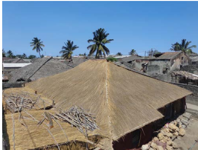
Fig. 11 An exemple of macuti house with renovated roof, using alternative grass coverage.
