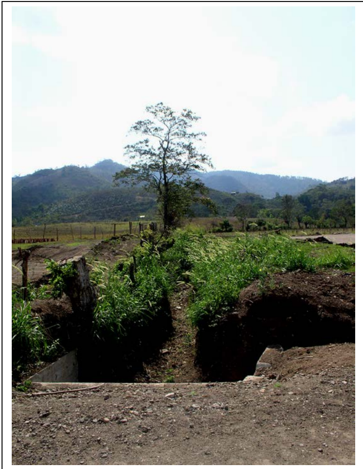
CURRENT WORKS AT LA ESTANZUELA FOR DRAINAGE SYSTEM.
