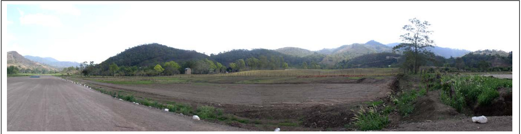
LA ESTANZUELA. NORTHEAST VIEW OF THE AIRSTRIP. CLEARED LAND ON THE LEFT IS FOR INFRASTRUCTURE CONSTRUCTION
