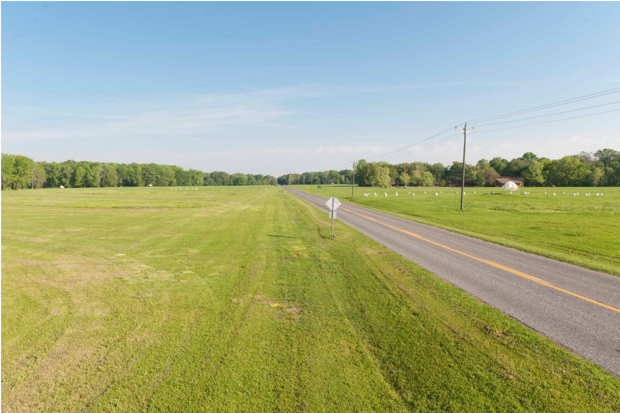
Figure 6. Highway 577 passing through Poverty Point World Heritage Site. Photo © C.C. Lockwood
