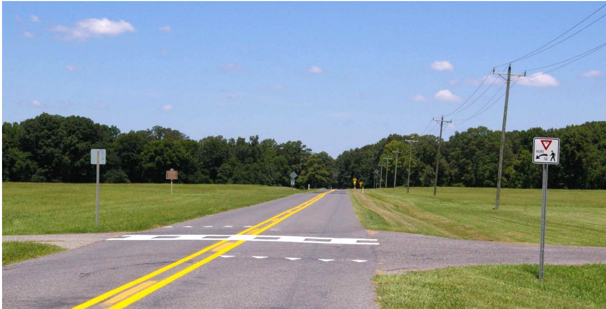
Figure 8. Refinished crosswalk with “shark’s teeth” yield lines and associated reinforcing yield sign at the northern crossing of the interpretive driving trail. Photo: Diana Greenlee
