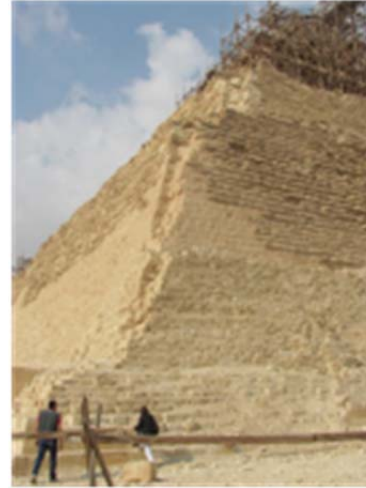
Fig. 4 – uncompleted south-east corner
