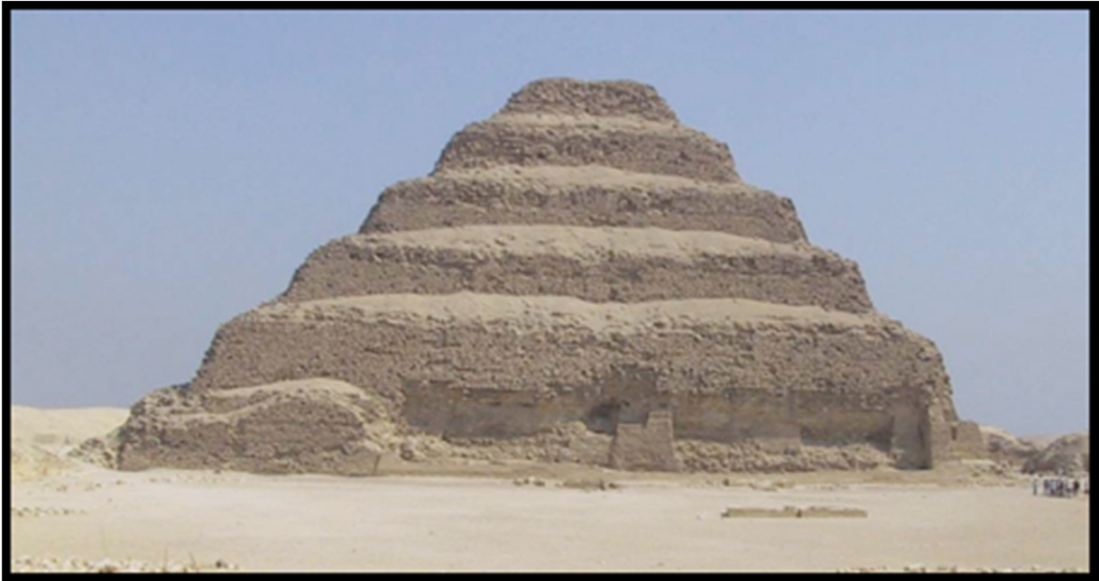
The Southern elevation of the Djoser Pyramid of Saqqara before the works (Photo, Hassan Fahmy)
