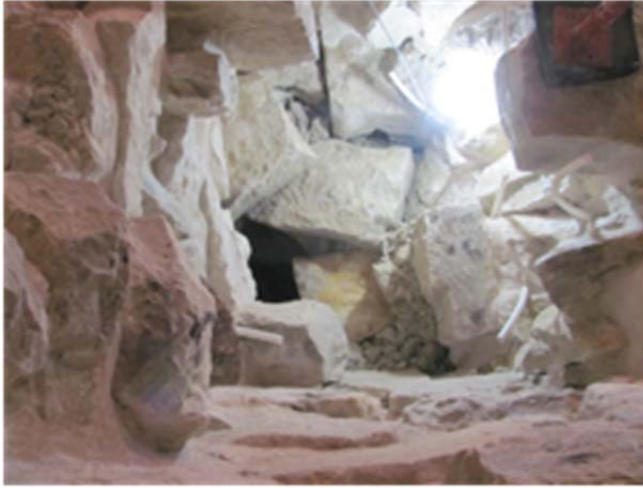
Fig. 3 – blocks in precarious conditions of stability
