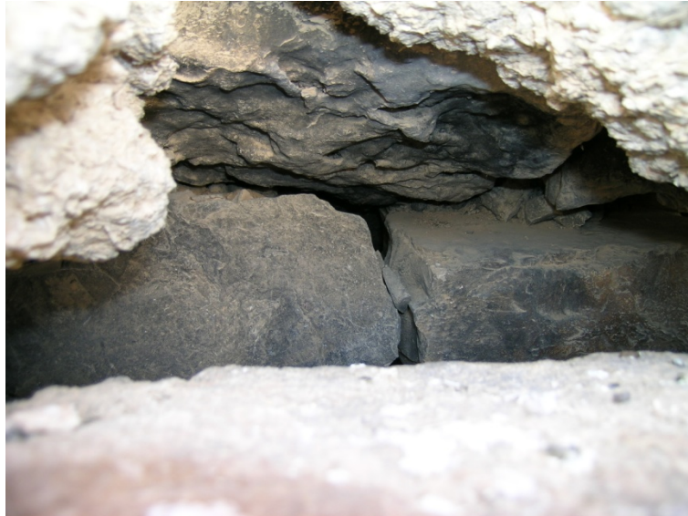
MASONRY INTERIEUR The interiors joints are hallow
