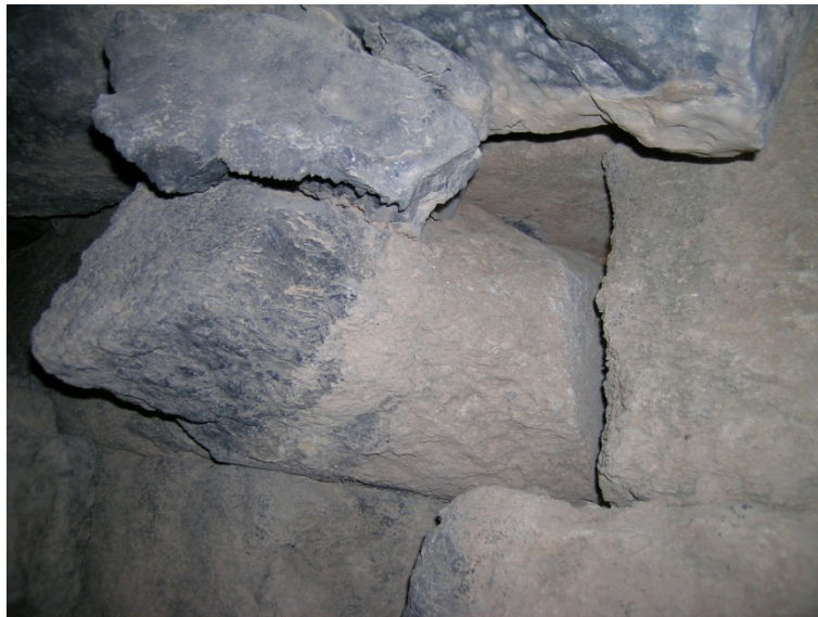
INSIDE THE BASIS OF THE TOUR A stone face is cut so as to stabilize the filling.
