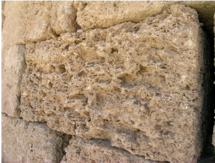
NORTH FACADE - Eroded stone.
