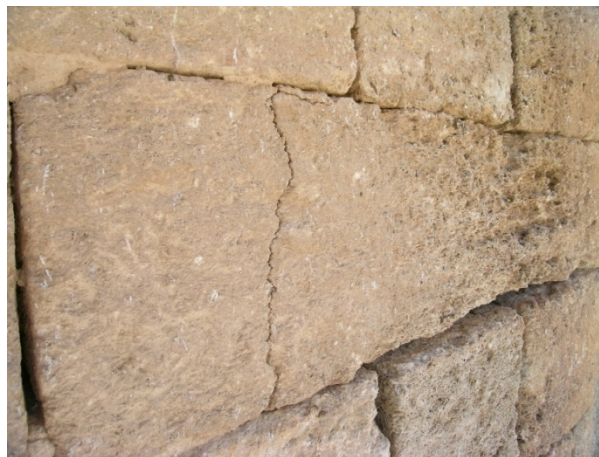
NORTH FACADE – Cracked stone.
