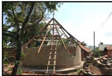
Walls and truss
