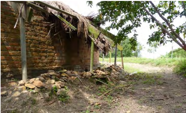
Back of the Tomb building. Water enters the building from all sides.
