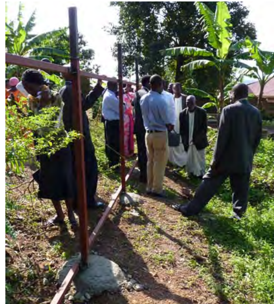
Steel frame of the security fence. The frame will be covered with reeds
