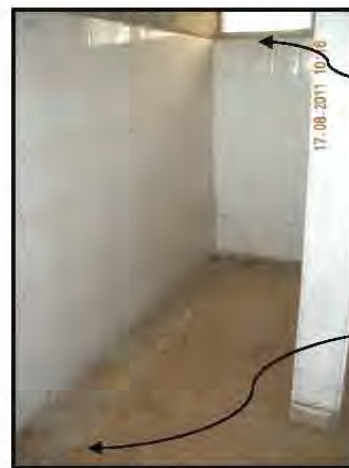
fig. 11c interior of the men's toilets, the tiles are in good condition, despite the dirt
