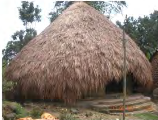
Fig. 8 'Abalongo Abasimbiri', structure still under construction
