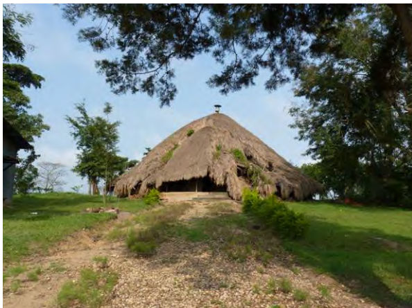
Front elevation of the tomb building (Batanda Bezaala)
