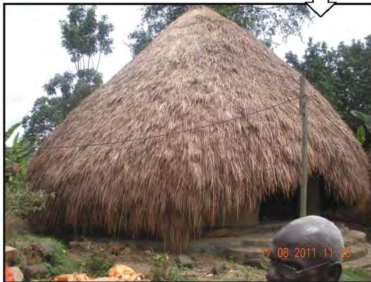
Thatching done: current status of the 'Abolongo Abasimbiri'
