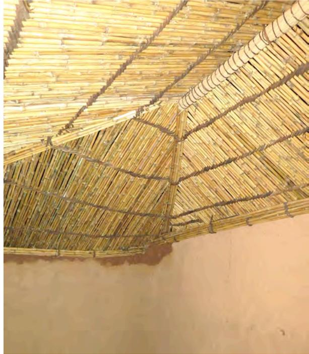
Top: Condition of the oldest surviving wattle-and-daub building on the site – the flat tin roof sheets arte original. Bottom: Repair of walls, roof trusses and inner thatch ceiling (Comparative photos S Moriset). Right: Detail of the roof repairs on the interior.
