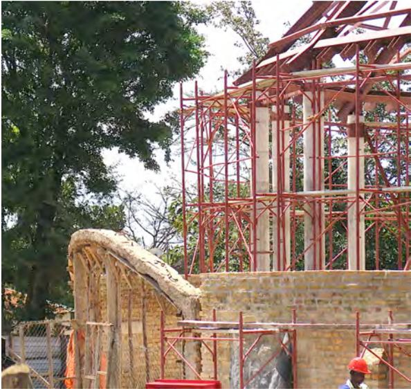
Detail of the concrete entrance portal damaged in the fire and to be rebuilt to adjust for the new roof pitch.
