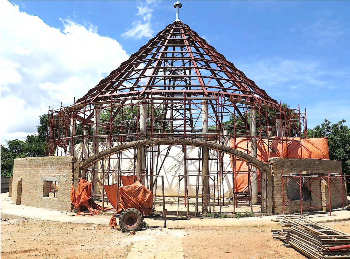
The *Muzibu-Azaala-Mpanga* of 1938 that is being reconstructed was a hybrid building with traditional thatching on timber beams and purlins and with inner rings of reeds and grass, timber columns and bark coverings and screens, but with a buttressed brick outer wall, and concrete columns and steel truss-work for the inner circle – the photograph provides the state of reconstruction on 13 May 2013,
