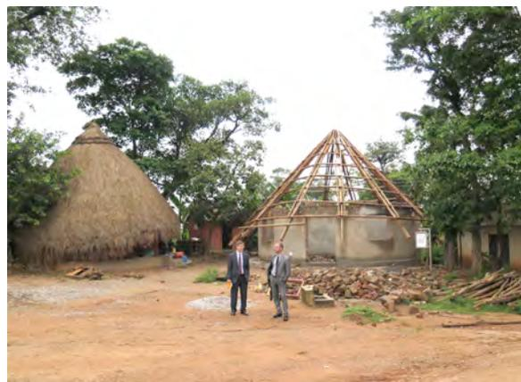
Metal roofs of inner ring houses are removed and replaced with roof poles and thatch.
