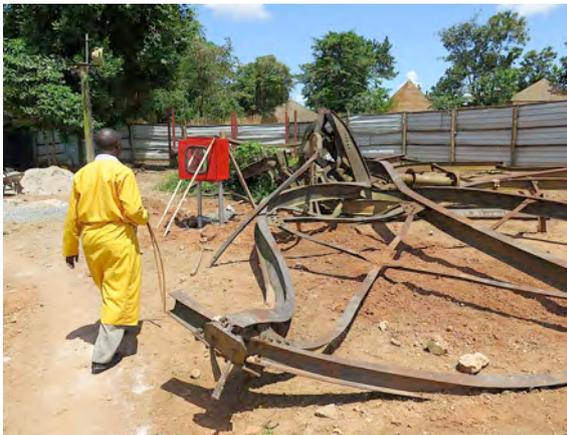
Remains of the 1938 steel roof truss-work burnt in the fire.
