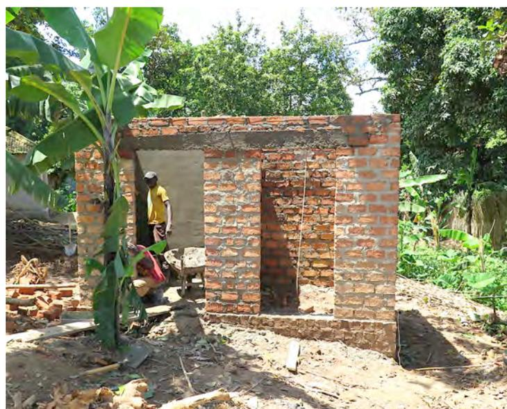
New cooking and ablation facilities in contemporary construction – brick, cement mortar, concrete floor and galv. monopitch sheet metal roofs.
