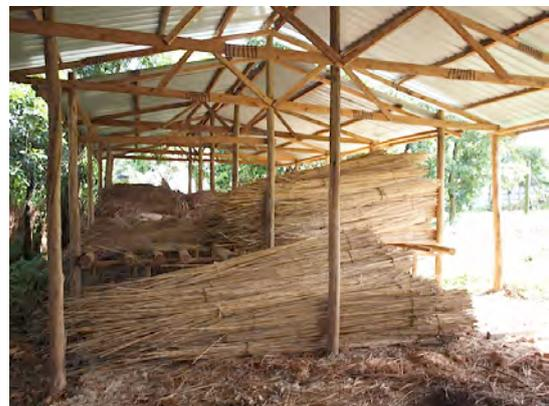
New roofed drying racks for thatching (This is a very large improvement on the site – however the thatch bundles are lying flat – research by Japanese experts shows that this method still causes moisture so drying cables/rods have to be installed).
