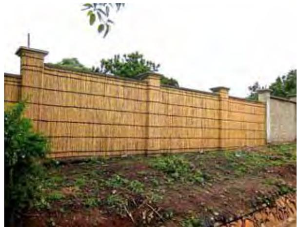
Left: newly constructed concrete block perimeter wall. Right: Cladding of wall and columns with reeds.
