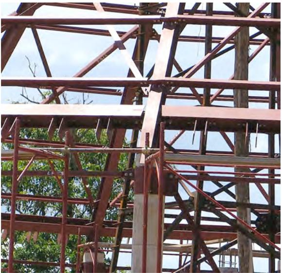
Detail of the steel truss-work of the inner circle roof with brackets to attach the timber beams of the lower roof.
