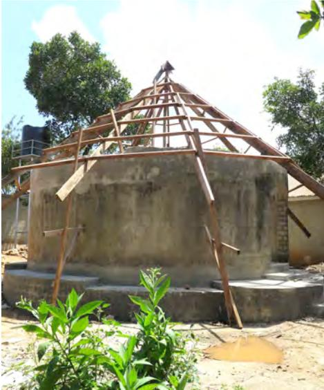
New concrete, brick and cement-plaster house with timber beams to be thatched.
