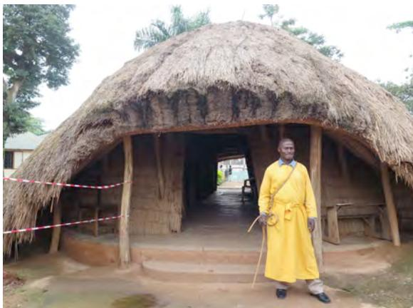
The gatehouse is leaning due to structural failure from termites. Documentation is complete and reconstruction is envisaged.
