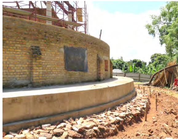
New outer paving to further prevent termite infestation.
