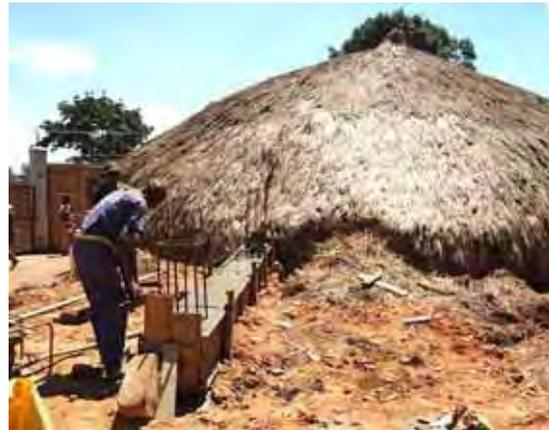
Right: New concrete inner wall abutting into thatch gate-house.
