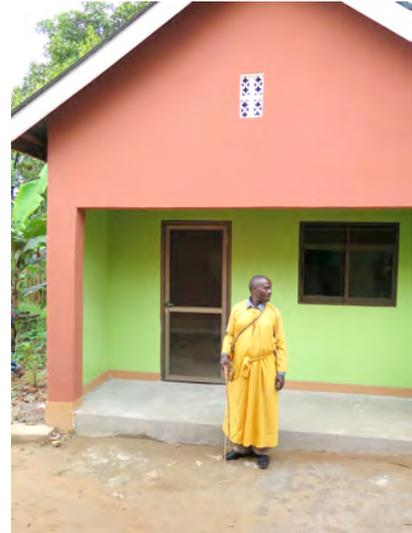
New tomb for royal wife - conventional concrete, brickwork and cement-plaster, with pitched saddle-roof aluminium window and door frames.
