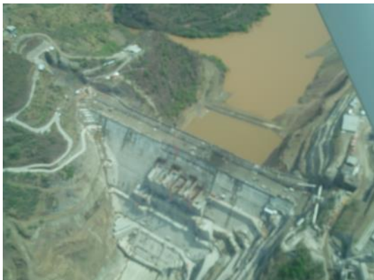
Picture 6: Gibe III dam. Photo © Edmond Moukala
