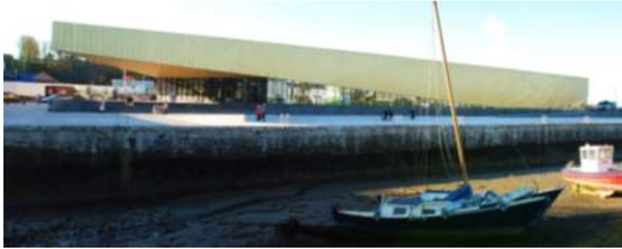
Note that the Fielden Clegg Bradley image above shows the greater impact of the bronze canopy in direct sun. Source: PowerPoint presentation 28 January 2015 by Mr Mike Keys and Mr Matt Williams of Fielden Clegg Bradley Architects.
