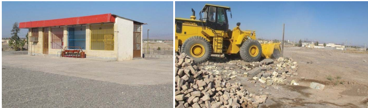
Figure 13. removal of non-adaptive structures
