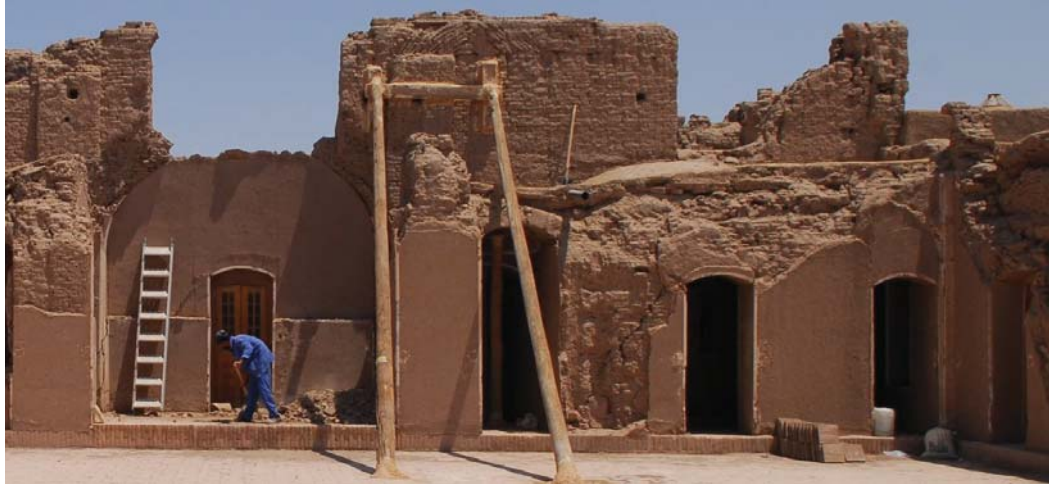
Figure 6. Restoration and conservation- Before outlining the main structure
