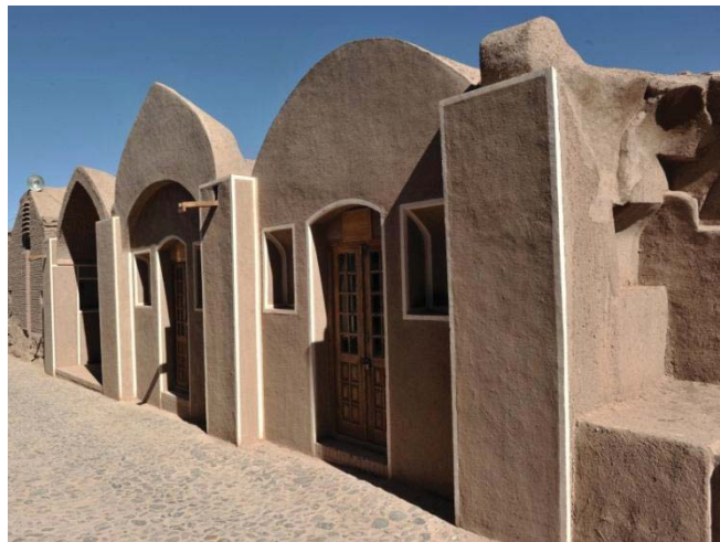
Figure 10. Rehabilitation of restored structures
