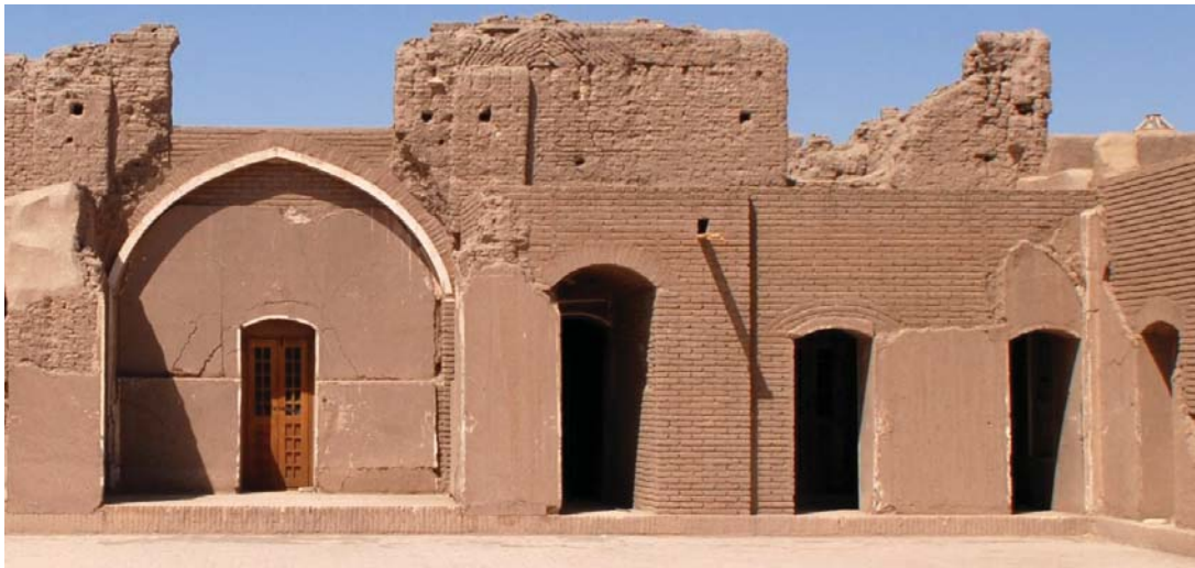
Figure 7. Restoration and conservation- After outlining the main structure
