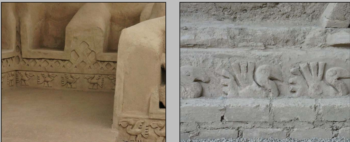
Figure 6. Covering of the ornaments with the fibreglass replicas (left) and with rows of adobes (right).
