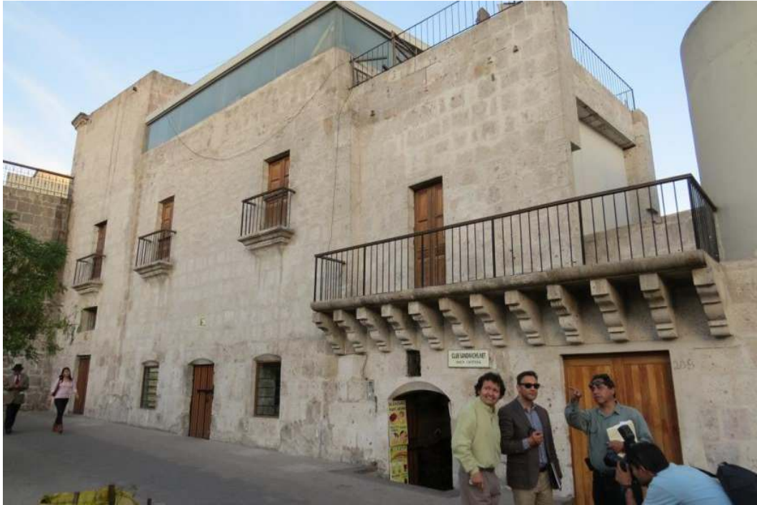
Restoration of Tambo La Cabezona with public housing.
