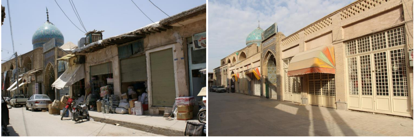
Figure 13. Masjed-e Ali passage- before and after reorganizing works
