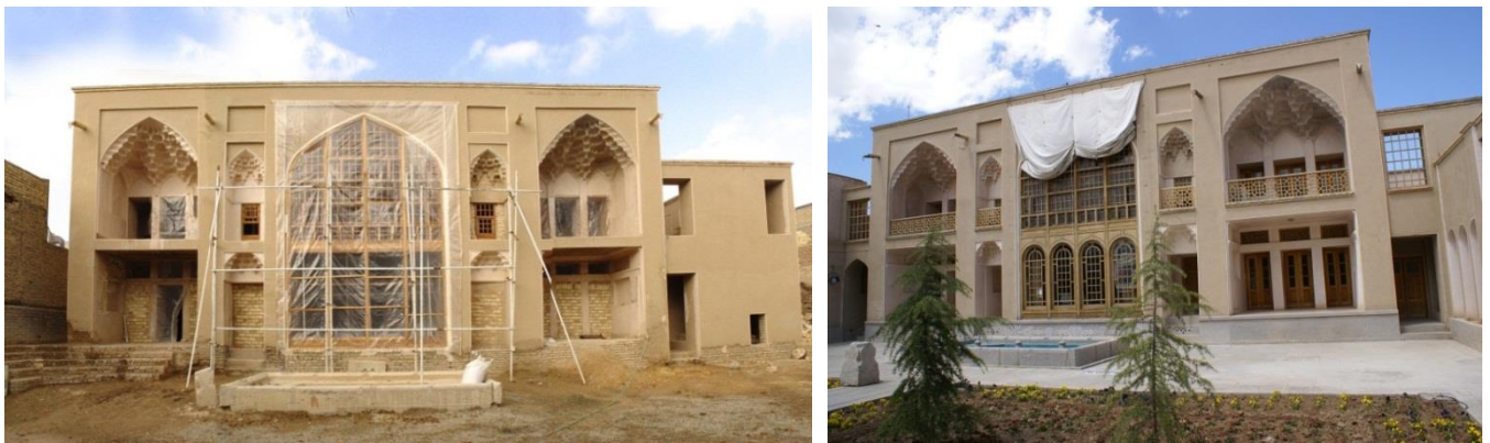
Figure 12. Harounye house- before and after restoration work
