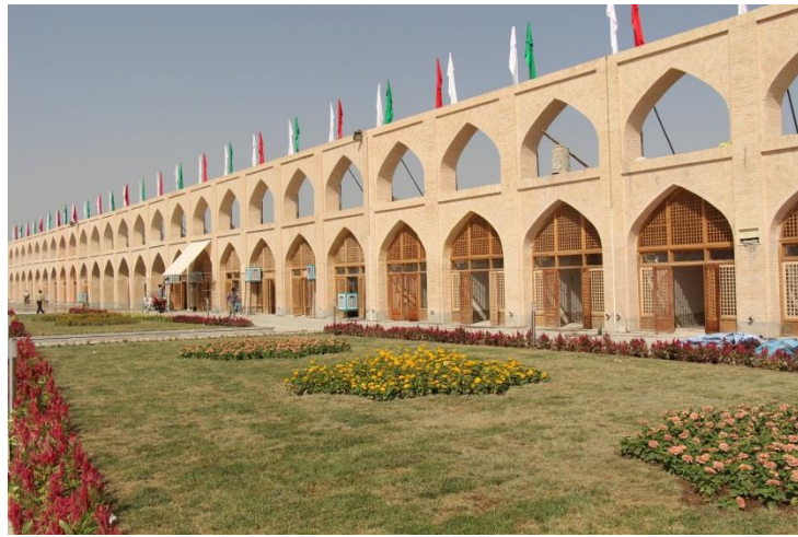
Figure 11. Western side of the Southern Section- Outcome of rehabilitation plan (right)
