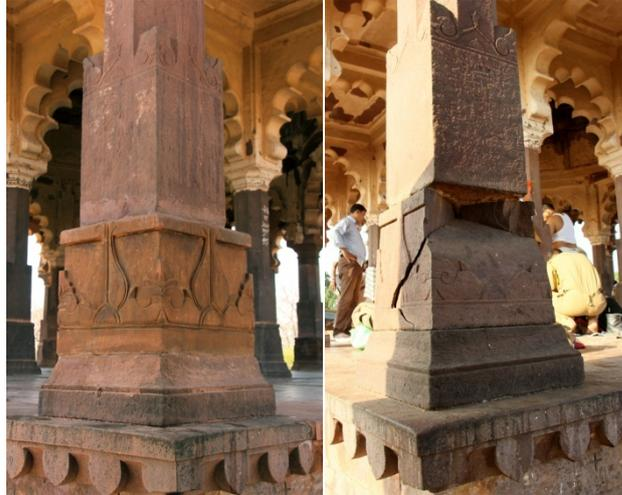
The broken base, shaft and capital of the stone pillars of Battish Khambha Chhatri have been taken up for conservation. The broken part is replaced with a new one, matching with the original. The broken/missing *pan*
