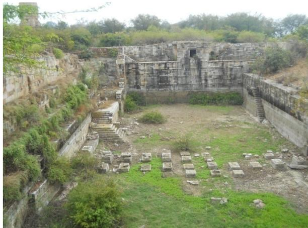
of vegetation through the masonry further leading to disintegration of the original structure. The floor of the reservoir was covered with 1 to 3 m debris consisting of silt and few architectural members. The ashlar masonry on the western arm was completely missing for about 3m on the top.
