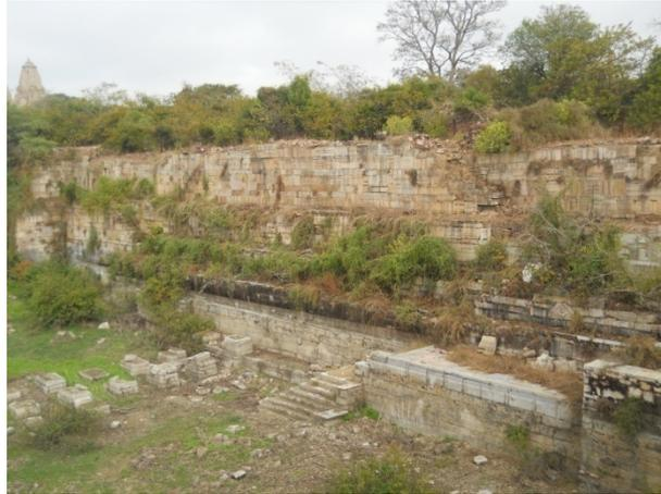
To begin with the accumulated debris on the floor of the reservoir is being cleared. Any architectural fragments and ashlar stones recovered from the debris will be reused appropriately. Further, conservation and restoration of the eastern arm to stabilise
