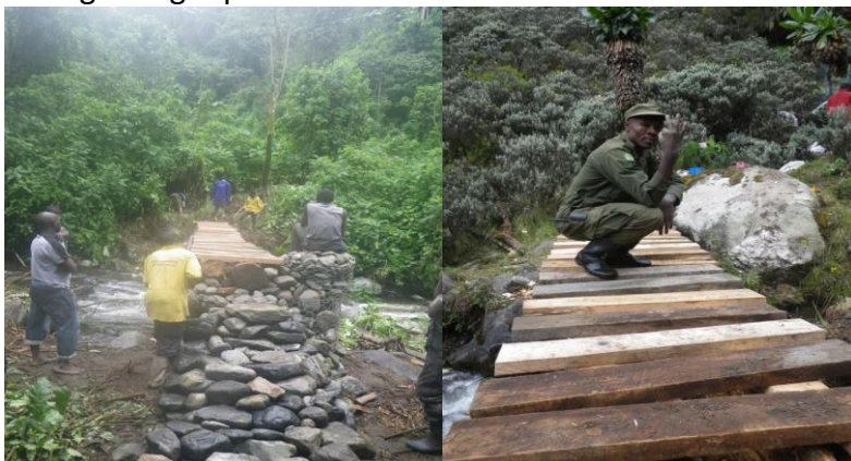
Access bridges on Kanywankoko and Bujuku rivers respectively after repair
