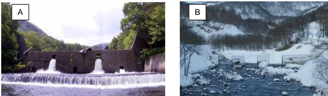
Fig. 10 Check dam before and after modification by making slits
