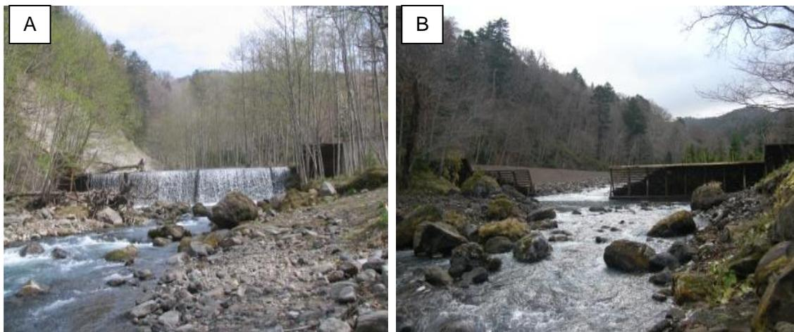
Fig. 6 Check dam before and after modification by making slits and lowering dam height
