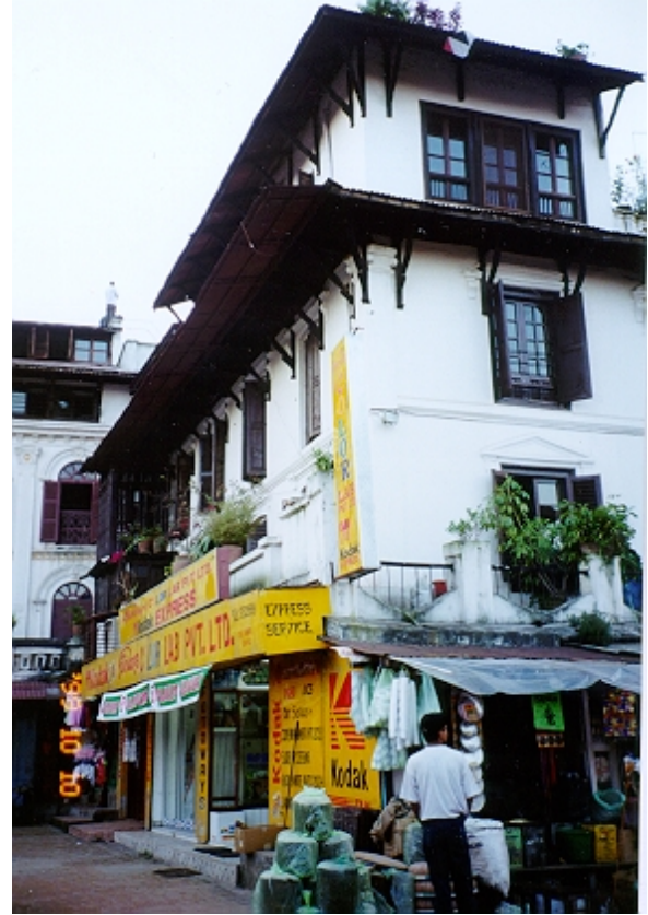
(Above) In October 1998, the original wooden shutters of this building, facing the Patan Darbar Square, were widened and replaced with metal shutters. Simultaneously, the entire ground floor was covered with inappropriate large bright advertisement which is illegal within the protected Monument Zones.
