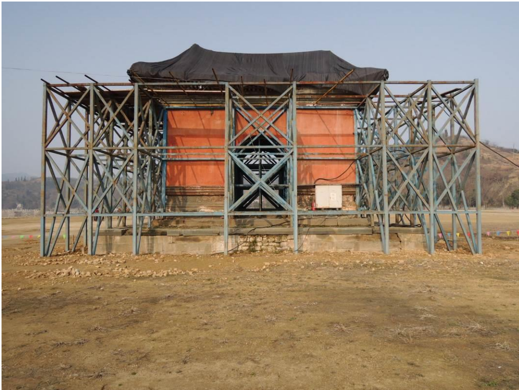
West Gate, Yuzhen Palace. One of three gates lifted up in situ . Photo: LD DiStefano
