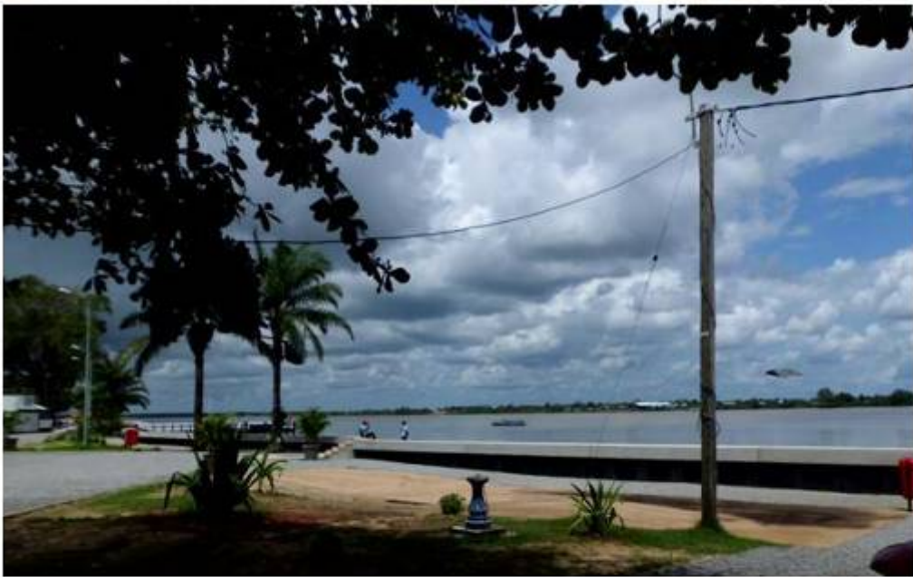
Views of the calm Waterfront and new seawall
