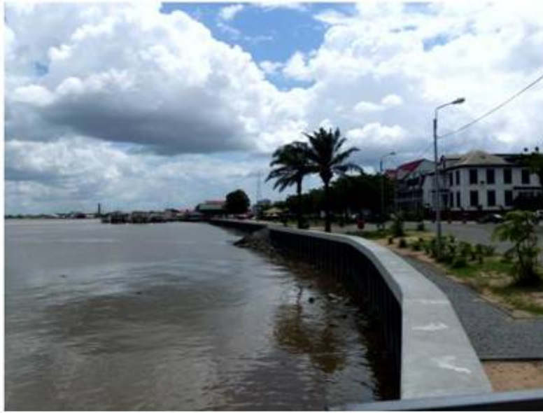
The seawall recently built
