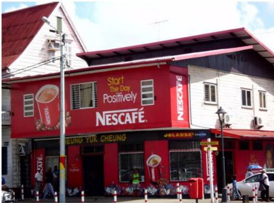
Inadequate painting and signs on the core zone
